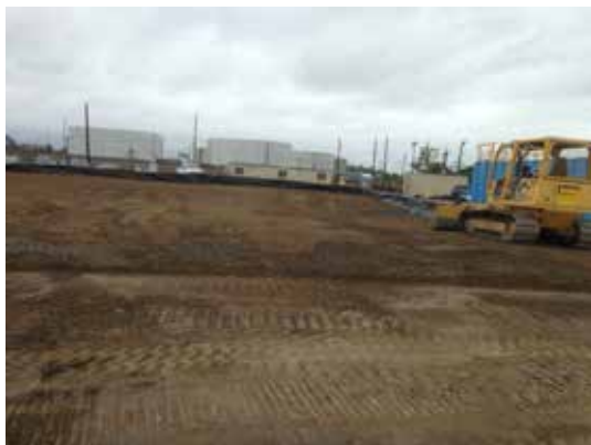
Compacting the ¾" AB on top of the geotextile
