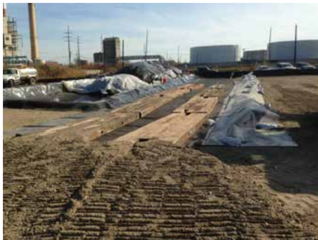
Crane mat road for the articulating dump truck
