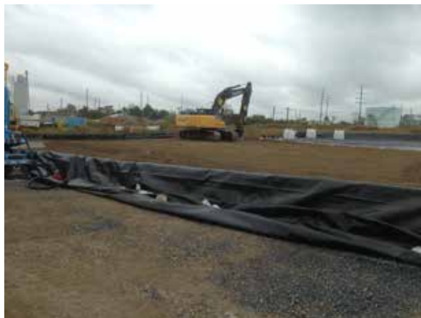
Placing ¾" AB on top of the geotextile
