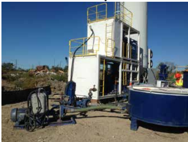
Connecting pumps to slurry plant
