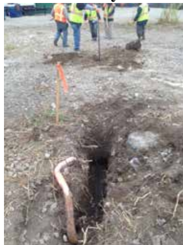
Hand digging to expose 2" pipe
