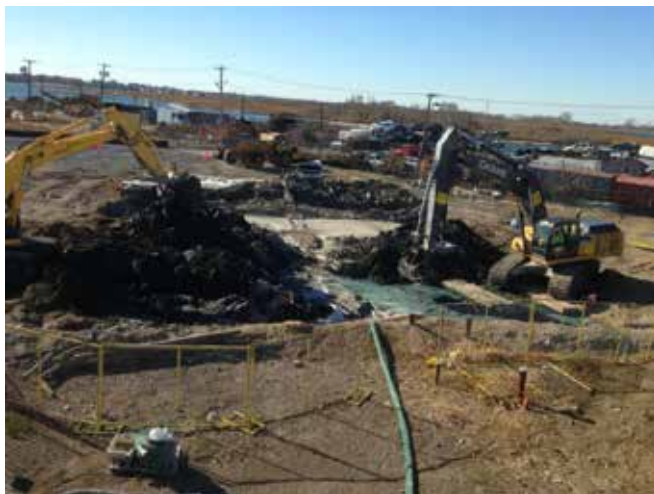
Mixing portland cement and loading out soils
