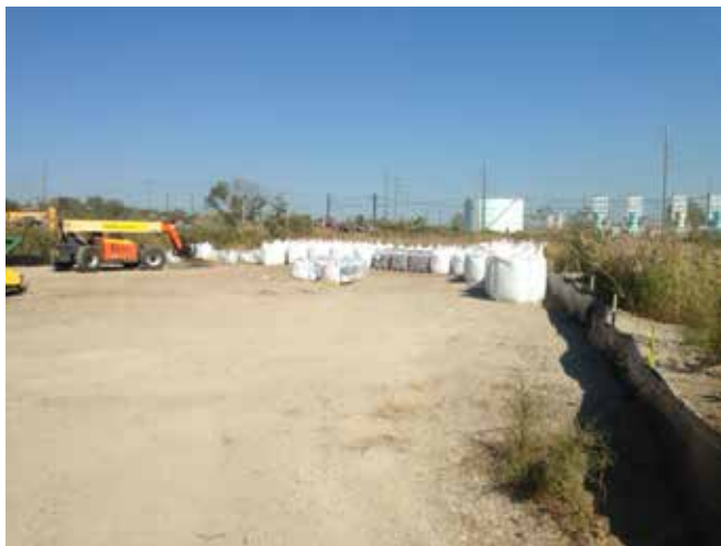
Bentonite delivered (48 total supersacks are on site)
