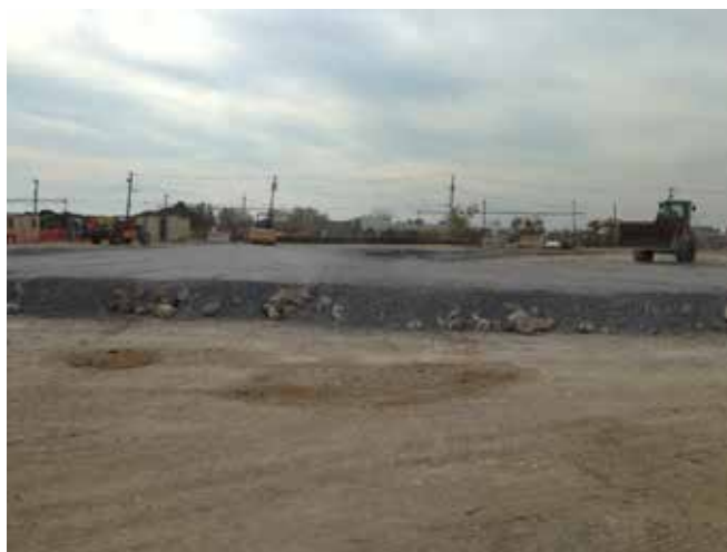
Grading SCA with \frac{3}{4} " rock
