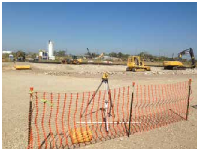
Rough Grading 1% fall for SCA
