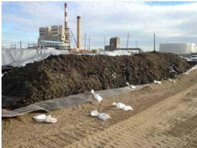
Moved materials out of excavation area to SCA
