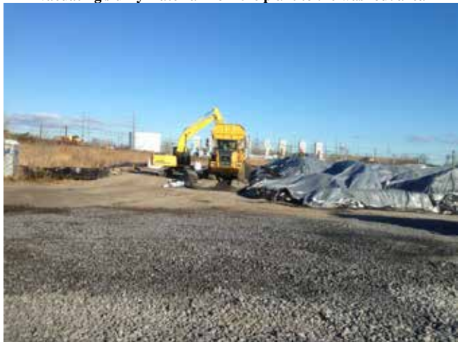
Evacuating slurry material from the plant to the washout area
