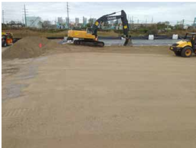
Compacting the ¾" AB on top of the geotextile
