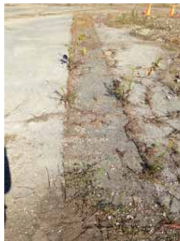
Saw cut patch along haul route
