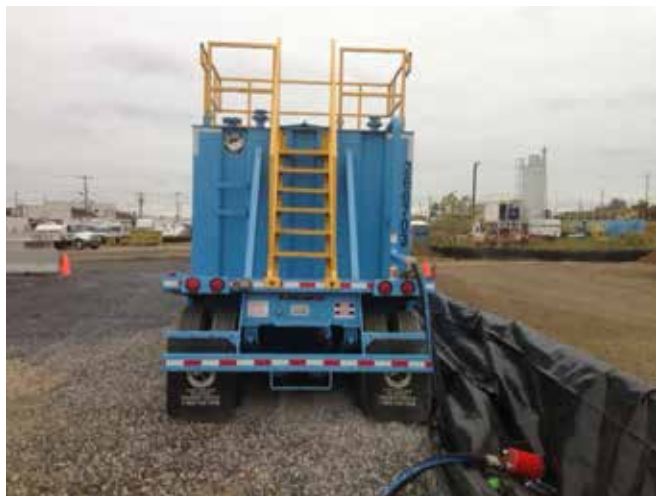
Preparing double wall frac tank connections
