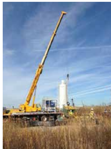
Crane picking up slurry tank
