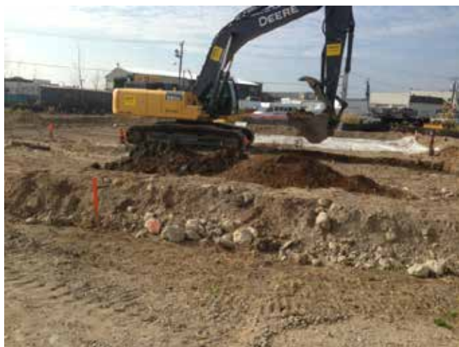
Upper 2' of soils removed from North end of Cell #1
