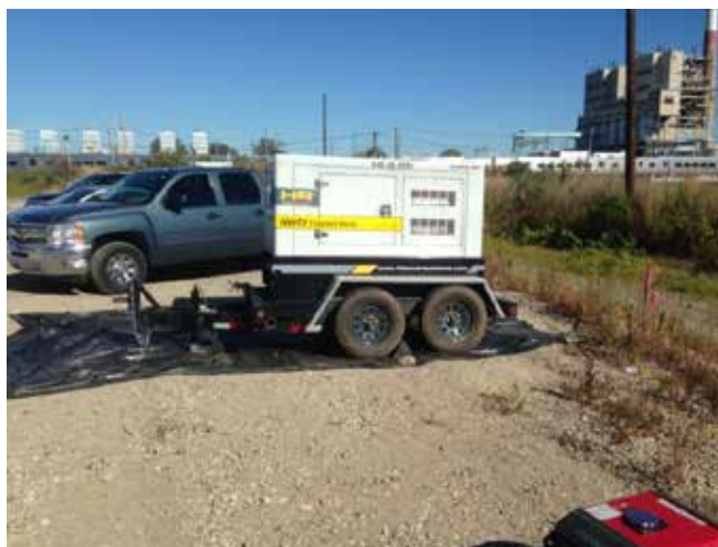
Setting up generator for connection to field trailer
