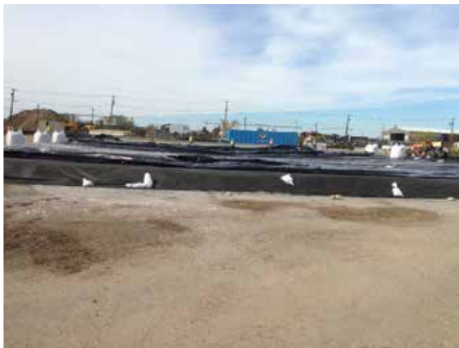
Anchoring liner with supersacks
