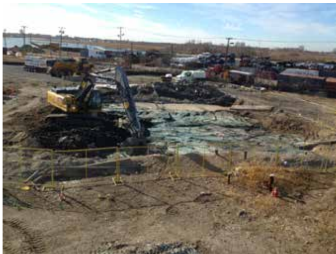
Loading out materials from the excavation area
