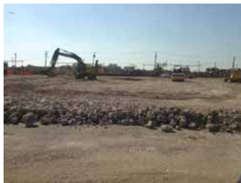
Rough Grading 1% fall for SCA
