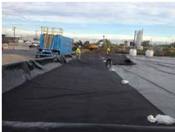
Placing 16oz geotextile on top of 40 Mil LLDPE liner
