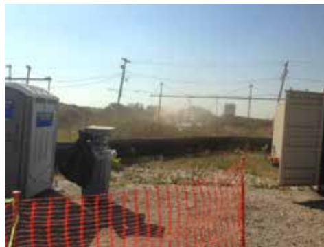
Bentonite delivered (48 total supersacks are on site)
