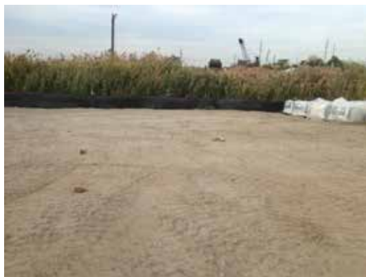
Grading SCA with \frac{3}{4} " rock
