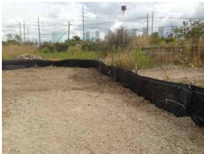
Silt fence completion
