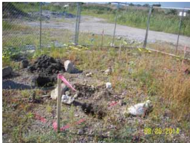
Hand-cleared areas of GS-2/GP-NORTH area to rule out utility.
