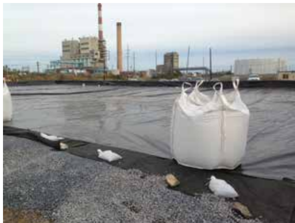
Placing geotextile and LLDPE liner
