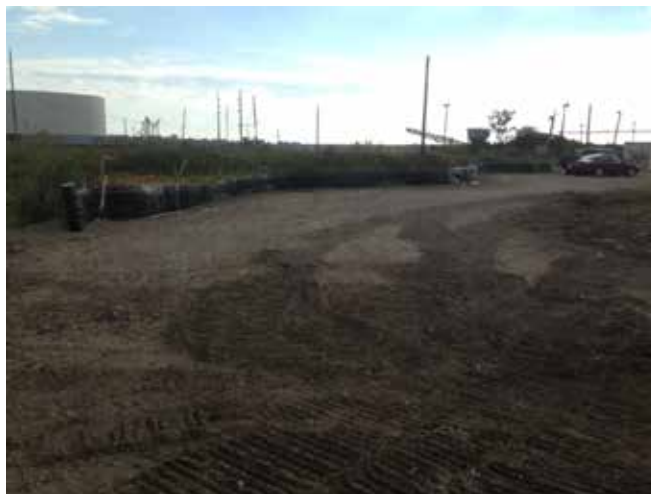
Silt fence installed
