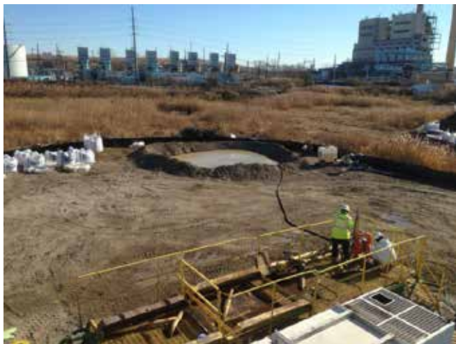
Evacuating slurry material from the plant to the washout area
