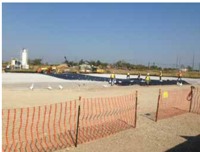
Geotextile installation
