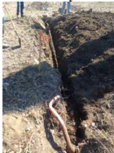
2'' pipe uncovered and ready to relocate/wrap
