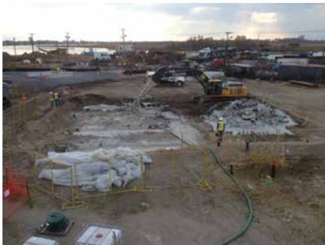
Excavation and CB slurry backfill of cell #5
