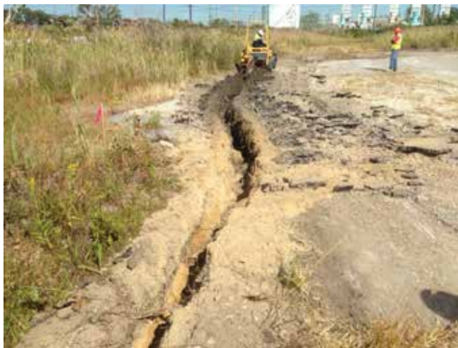
Silt fence trench
