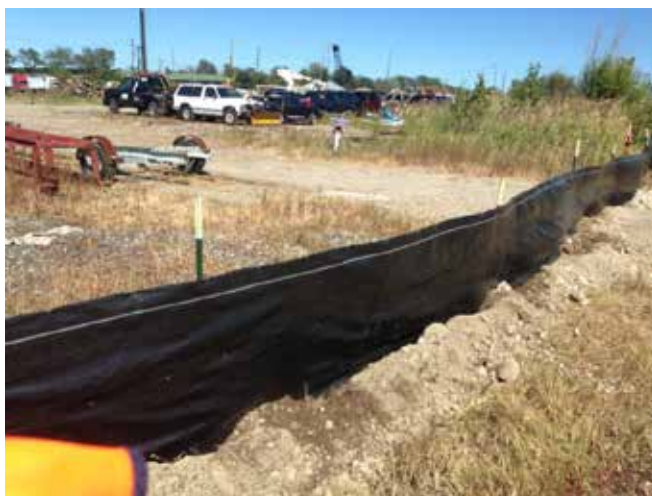
Installing silt fence along northern edge
