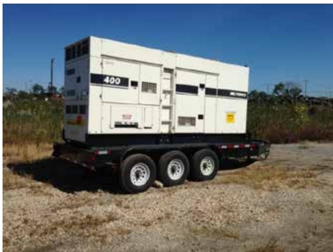
Generator for Slurry Plant
