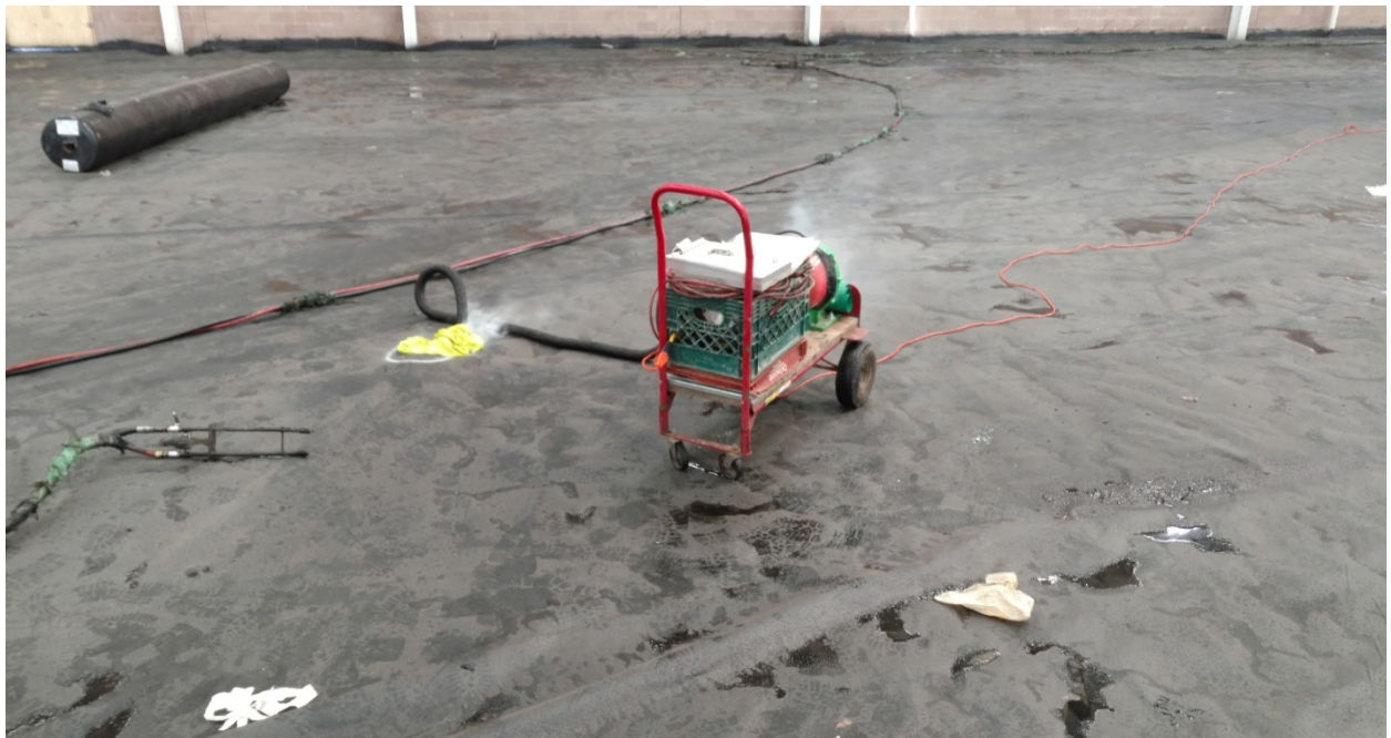
Photo #2: Depicts smoke testing of Liquid Boot Membrane.
