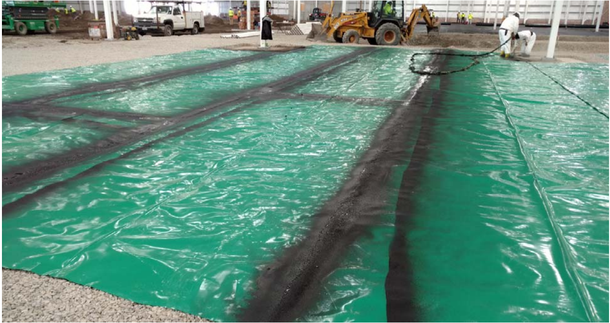
Photo #1: Depicts installation of vapor barrier system.
