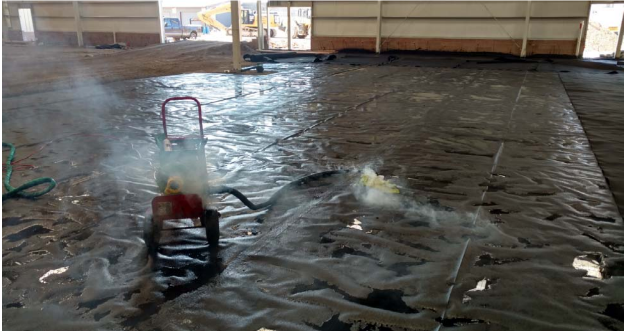
Photo #3: Depicts smoke testing of Liquid Boot Membrane.
