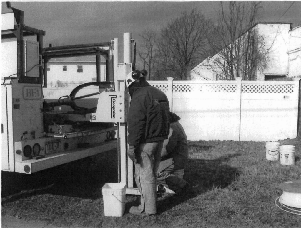
Photograph No. 3: Groundwater sampling activities.
