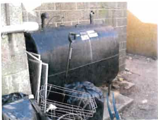
2. Rear yard area to north of building.
