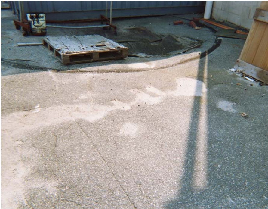
PHOTO 55: Depression area located near the northeast corner of the Global Pottery building at 301 Winding Rd.
