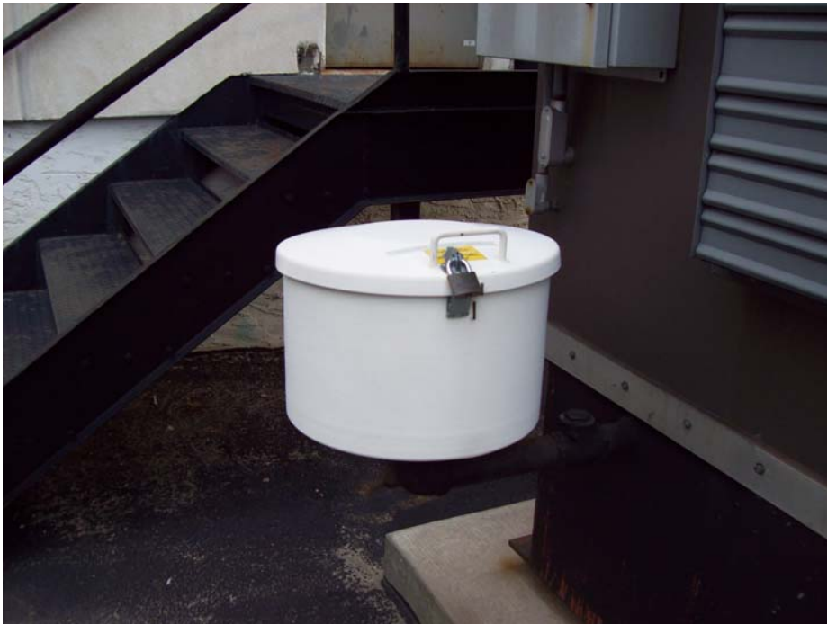
PHOTO 137: Diesel fuel fill port for AST, Arrow Electronics at 25 Hub Drive.
