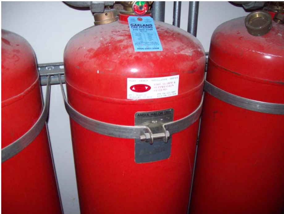
PHOTO 140: Tanks containing Ansul Halon 1301 which is part of the fire suppression system used in the Arrow Electronics building at 25 Hub Drive.
