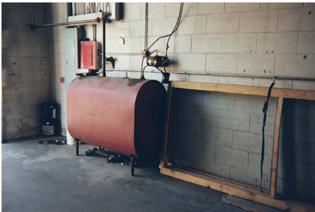
PHOTO 18: One of two ASTs that had contained #2 fuel oil in the National Maintenance, Inc. building at 175 Bethpage-Sweethollow Rd. Tanks have not been used since National Maintenance, Inc. has been a tenant.
