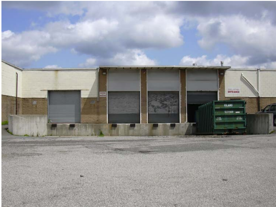
Photo 12: Loading area. Rear of building.
