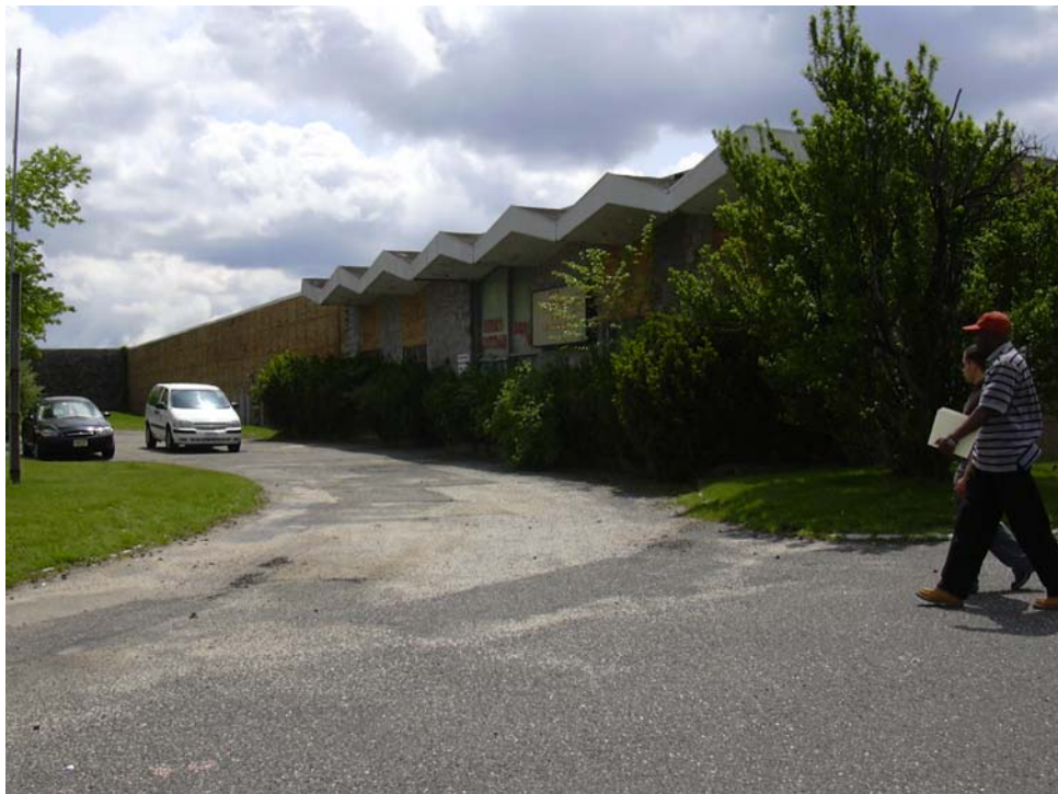
Photo 18: Front entrance 601 Cantiague Rock Road
