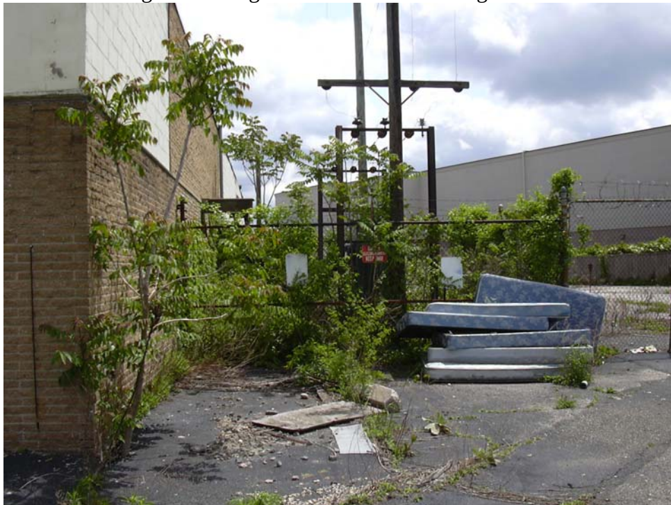
Photo 16: Transformer area. Rear wall, west corner. 601 Cantiague Rock Road
