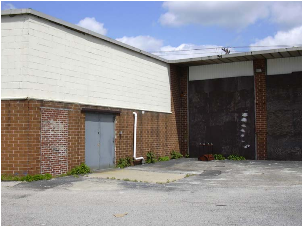
Photo 8: Loading area. Rear of building.
