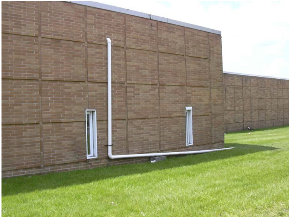
Photo 4: View of north walls where buildings adjoin (601 and 603 Cantiague Rock Road)
