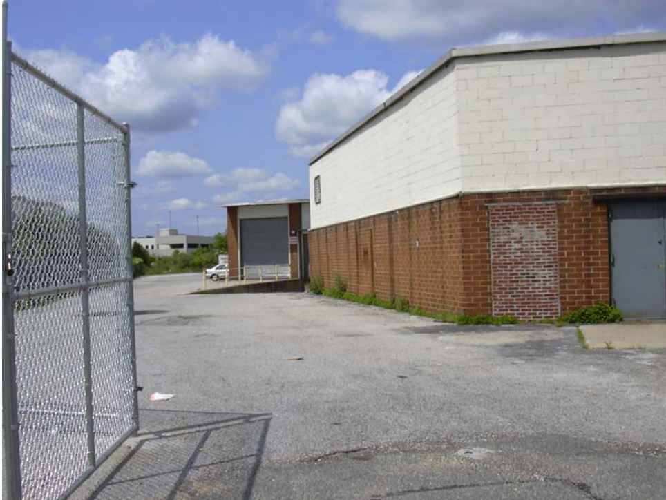
Photo 7: View of rear wall (loading area) 603 Cantiague Rock Road
