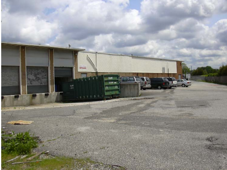
Photo 13: Loading area. Rear of building.
