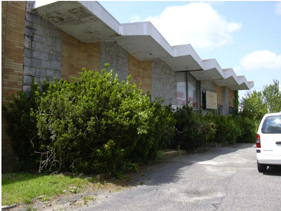
Photo 2: Front entrance 601 Cantiague Rock Road
