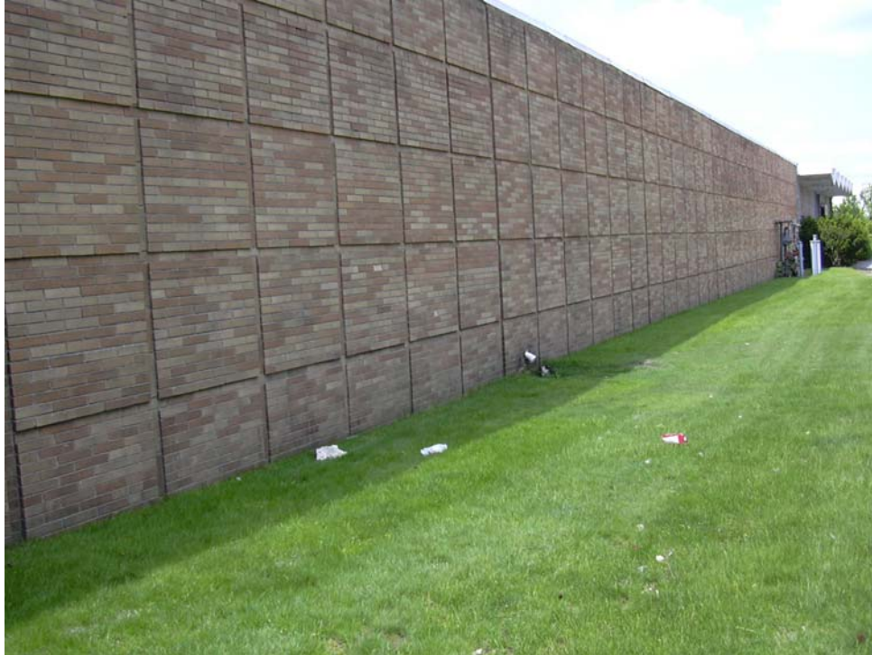
Photo 3: View looking at west along front entrance 601 Cantiague Rock Road
