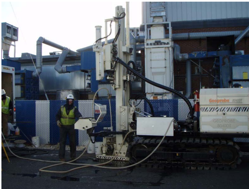
Geoprobe 8040 Rig for Hydropunch Well Installation
