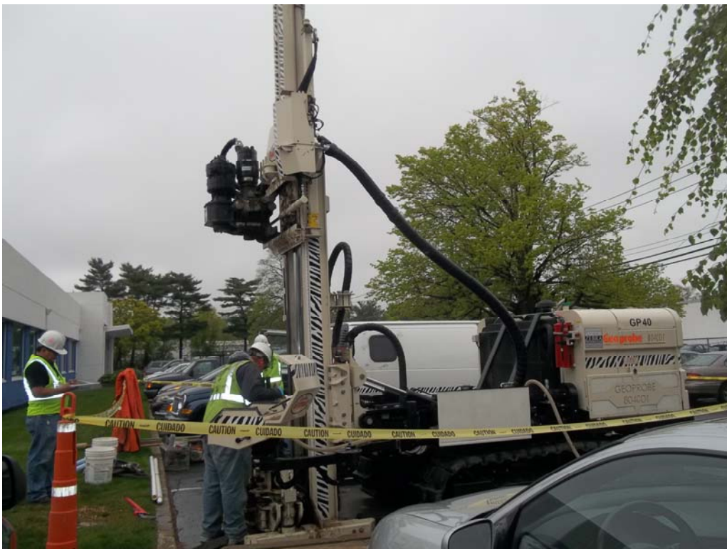
Permanent Well Installation with Direct Push Rig
