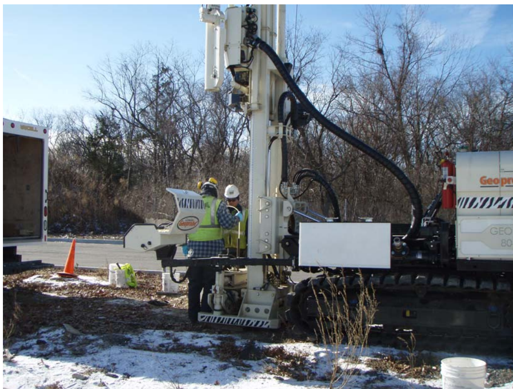
Hydropunch Well Installation at Sample Location DPW-W
