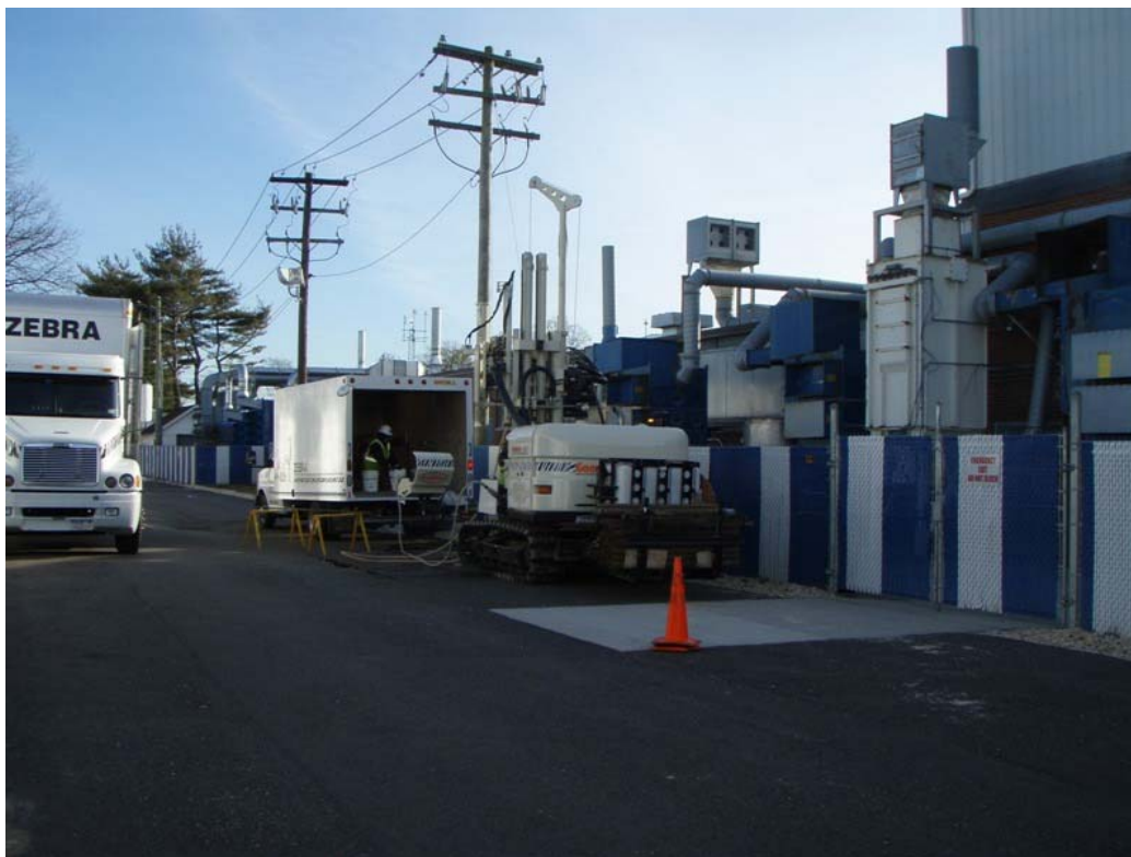
Hydropunch Well Installation at Sample Location BOC-C
