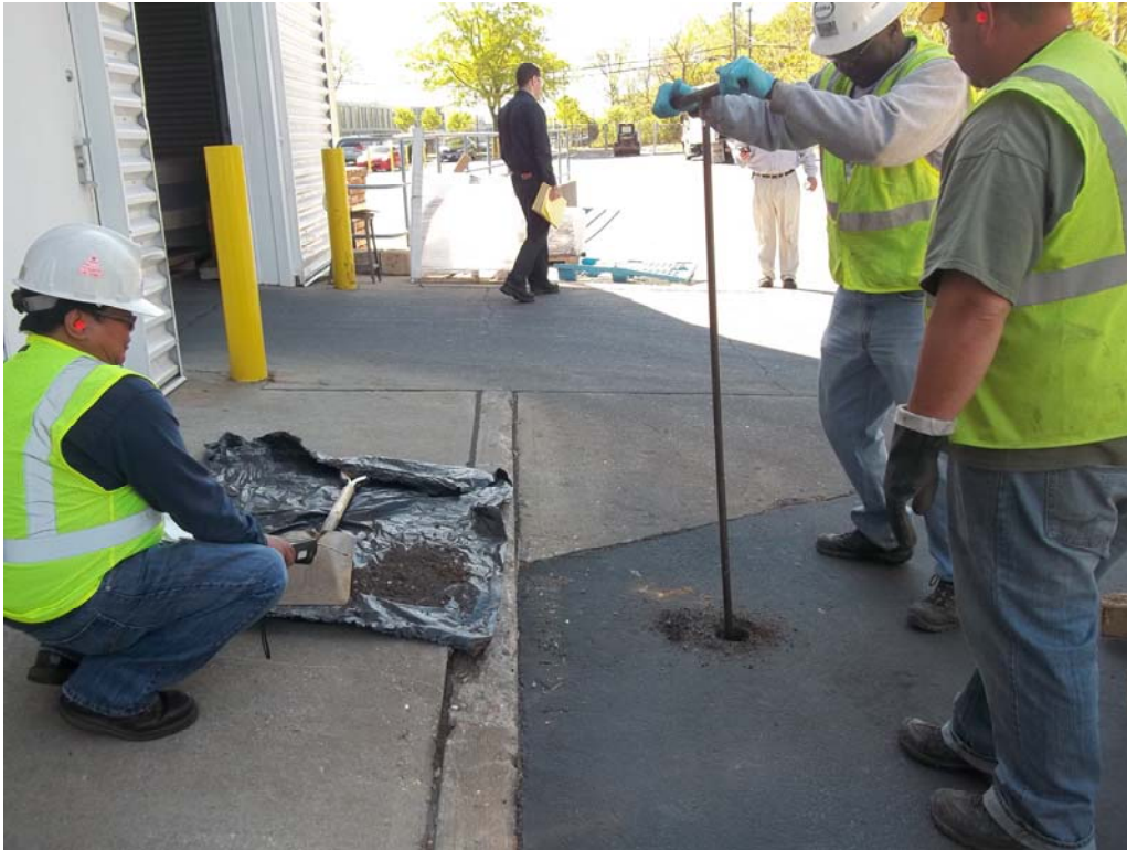
Hand Clearing Borings on Sulzer Metco, Inc. Property
