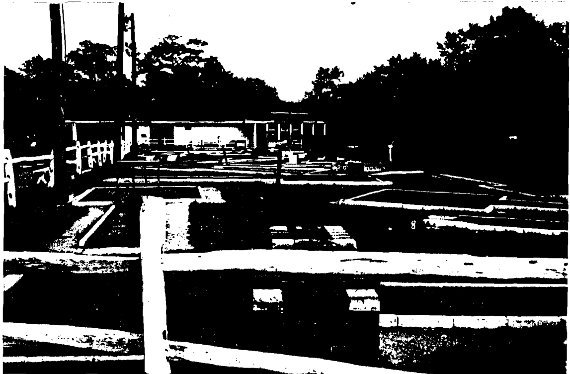
#2- Picture showing southeast corner of site (miniature golf/driving range).
