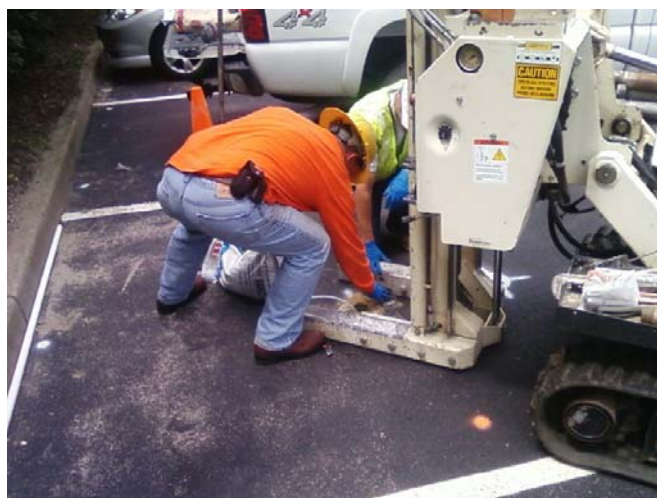
Installing Vapor Point.
