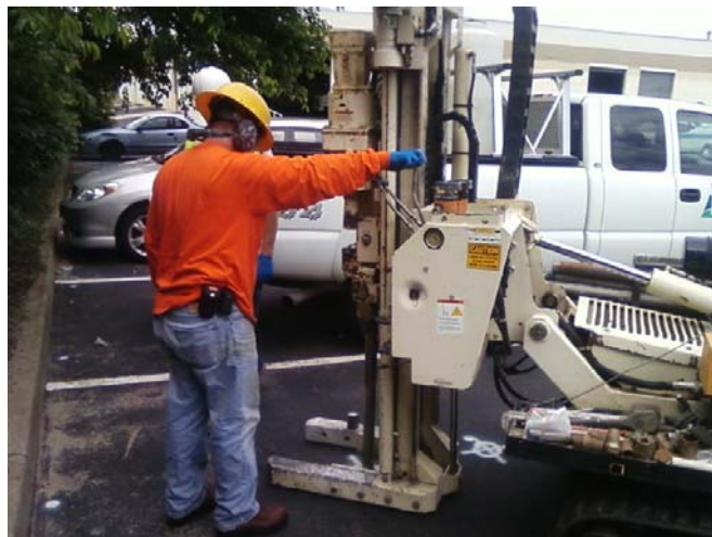
Geoprobe Drilling
