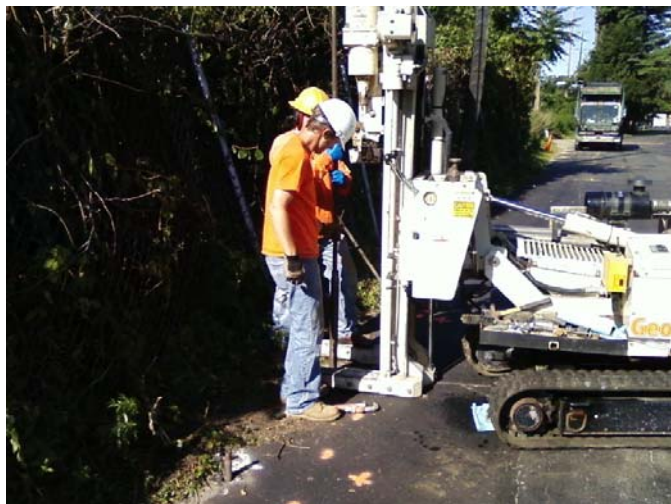
Installing hydropunch and drive rods
