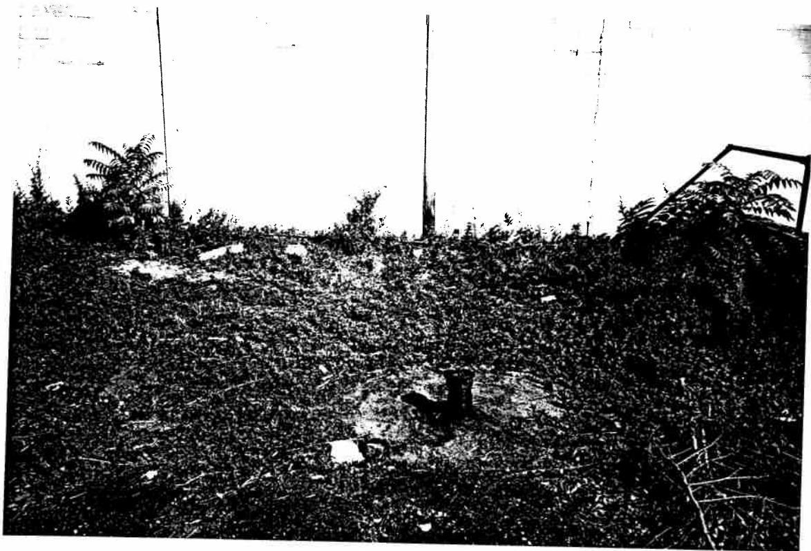
Fill pipe for 20,000 gallon fuel oil tank south of Building 10.
