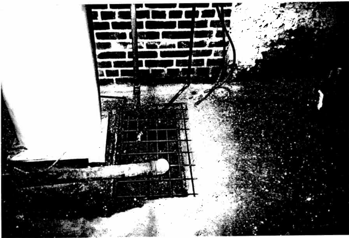
Floor drain in Building 7 that recieves compressor blowdown.
