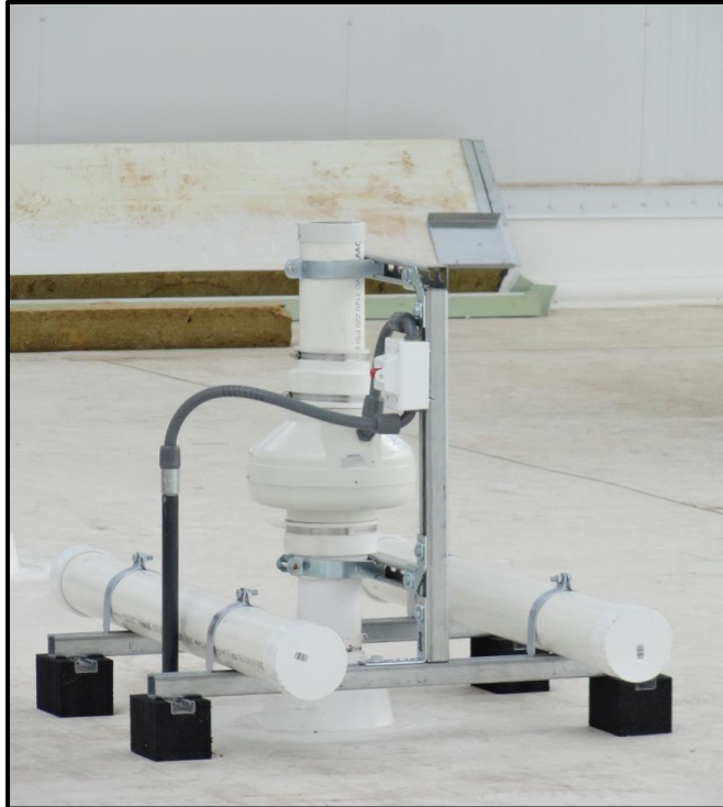
Roof Mounted Inline Centrifugal Blower
