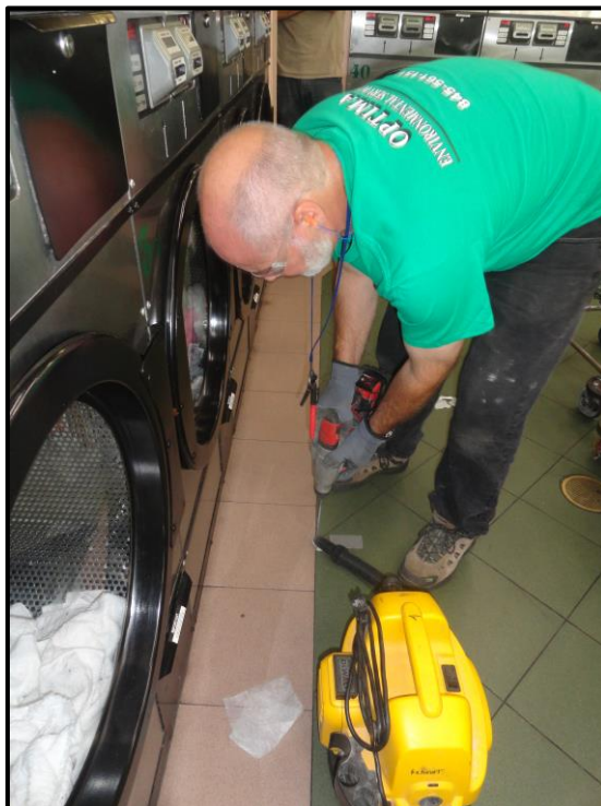
Drilling Remote Pressure Differential Measuring Holes
