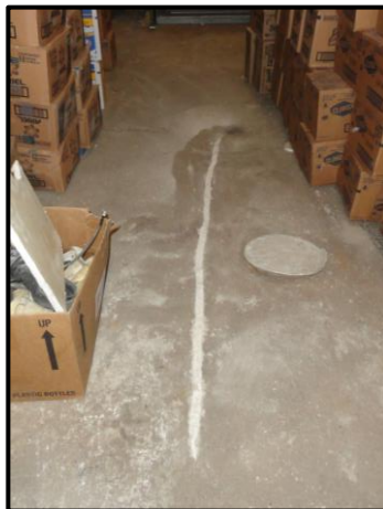
Water Channel Cut to Floor Drain
