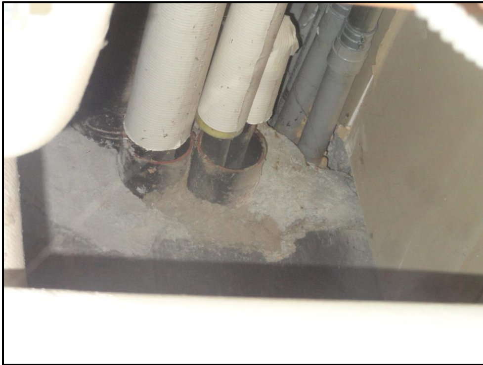
Conduit Openings to be Sealed
