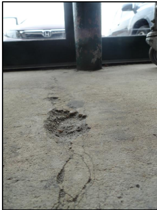
Floor Cracks to be Sealed
