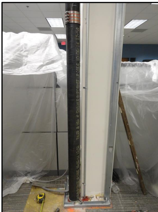
Metal Pipe Through Second Floor to Roof
