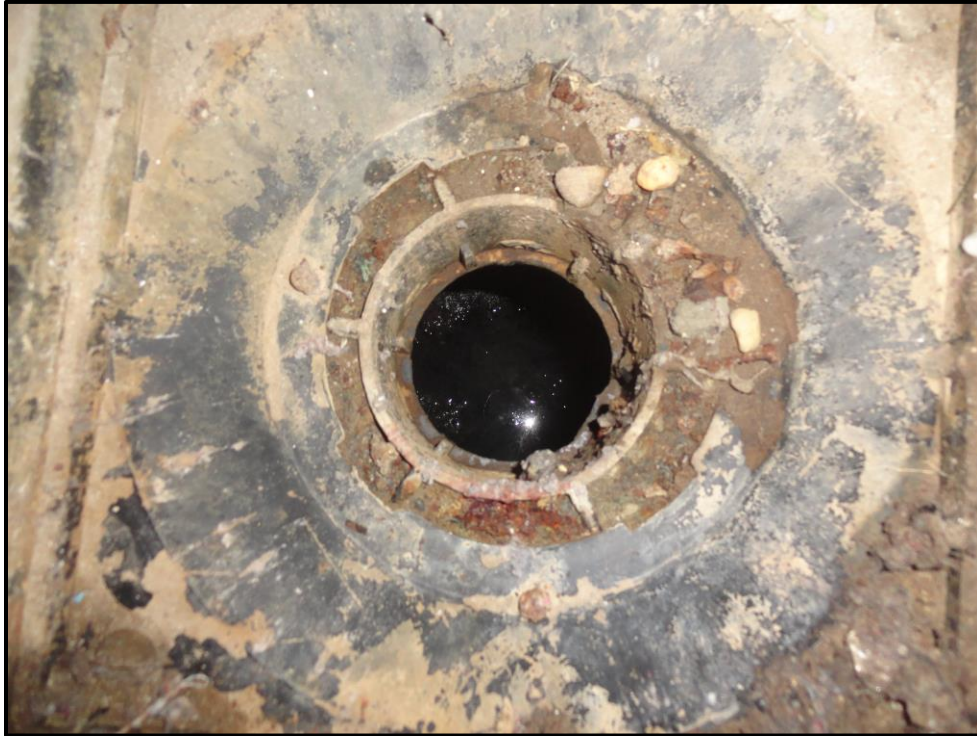
Underground Drainage Vault to be Sealed with a One Way Valve
