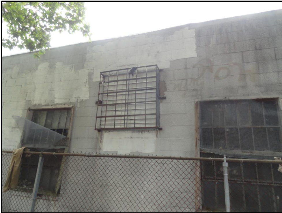
Open Windows and Louvered Wall Vent to Provide Continuous Passive Supply Venting to Replace Air and Exhaust by the Dryers
