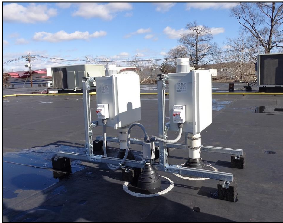
Roof Mounted Compact Radial Blowers
