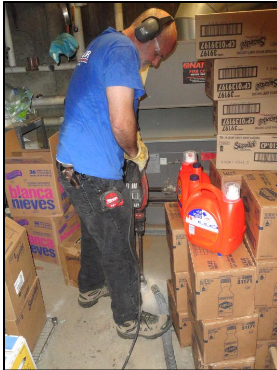
Coring Primary Diagnostic Suction Hole
