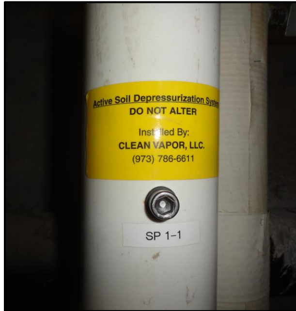
System Labeling and Test Port on a Riser Pipe
