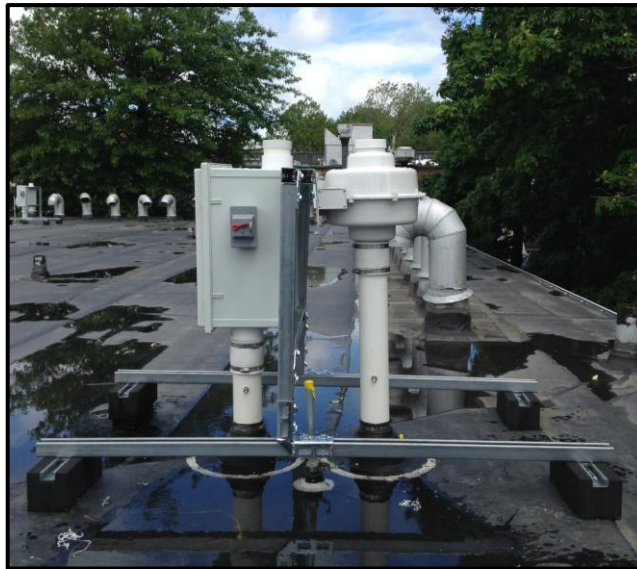
Roof Mounted Blower #1 and Blower #2
