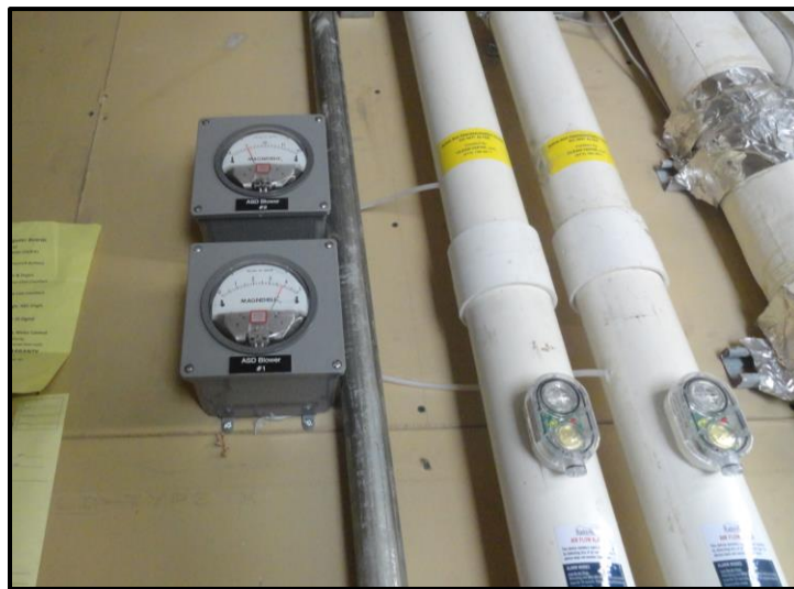
Magnehelics and RadonAway Air Flow Alarm
