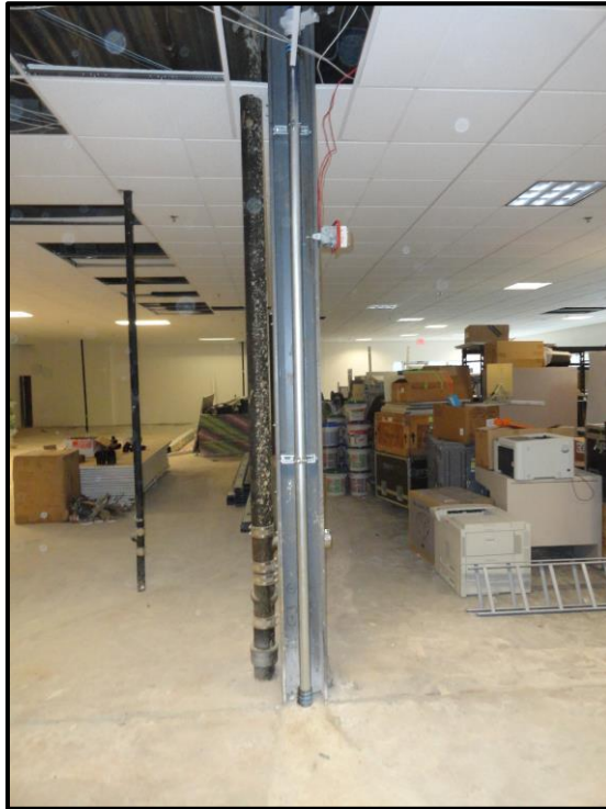
Suction Point and Metal Riser Pipe
