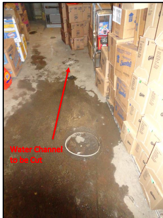
Bucket and Exposed Soil to be Removed and Sealed with Concrete Water Channel to be Scored into Concrete Floor in the Direction of the Floor Drain
