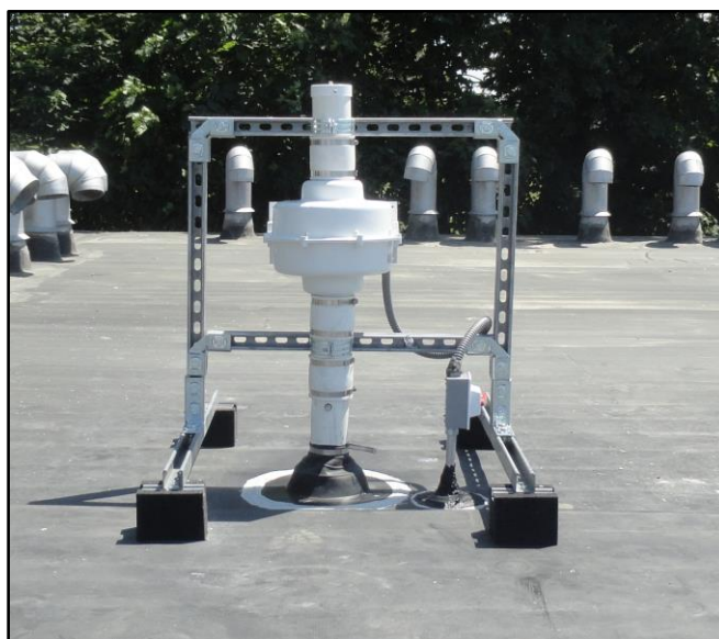
Roof Mounted Blower # 3
