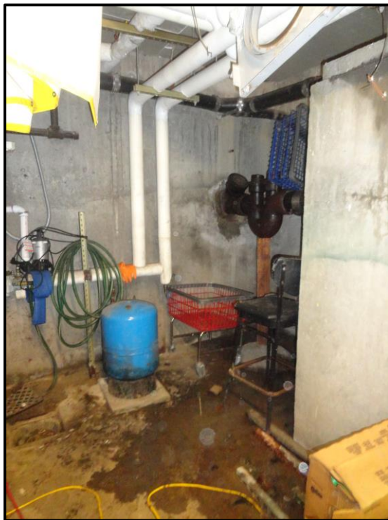
Waste Water Wash Lint Separator Overflowed While We Were Onsite. This Assembly Requires Scheduled Servicing.
