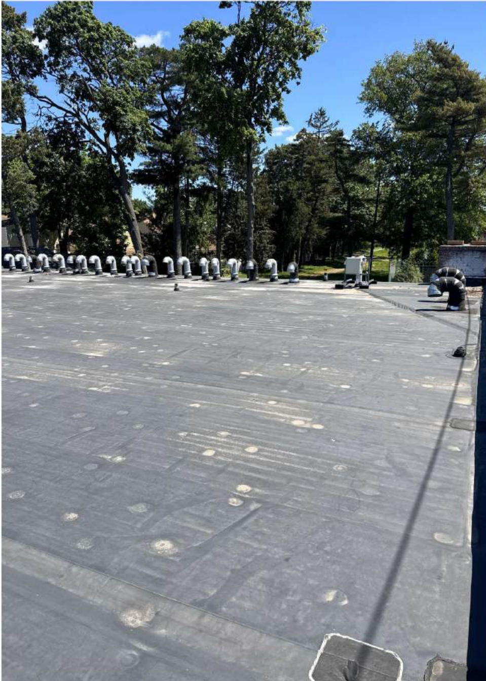
Roof Looking East
