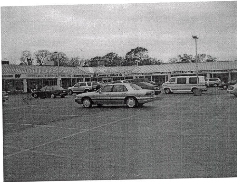
1. View of the subject building.
