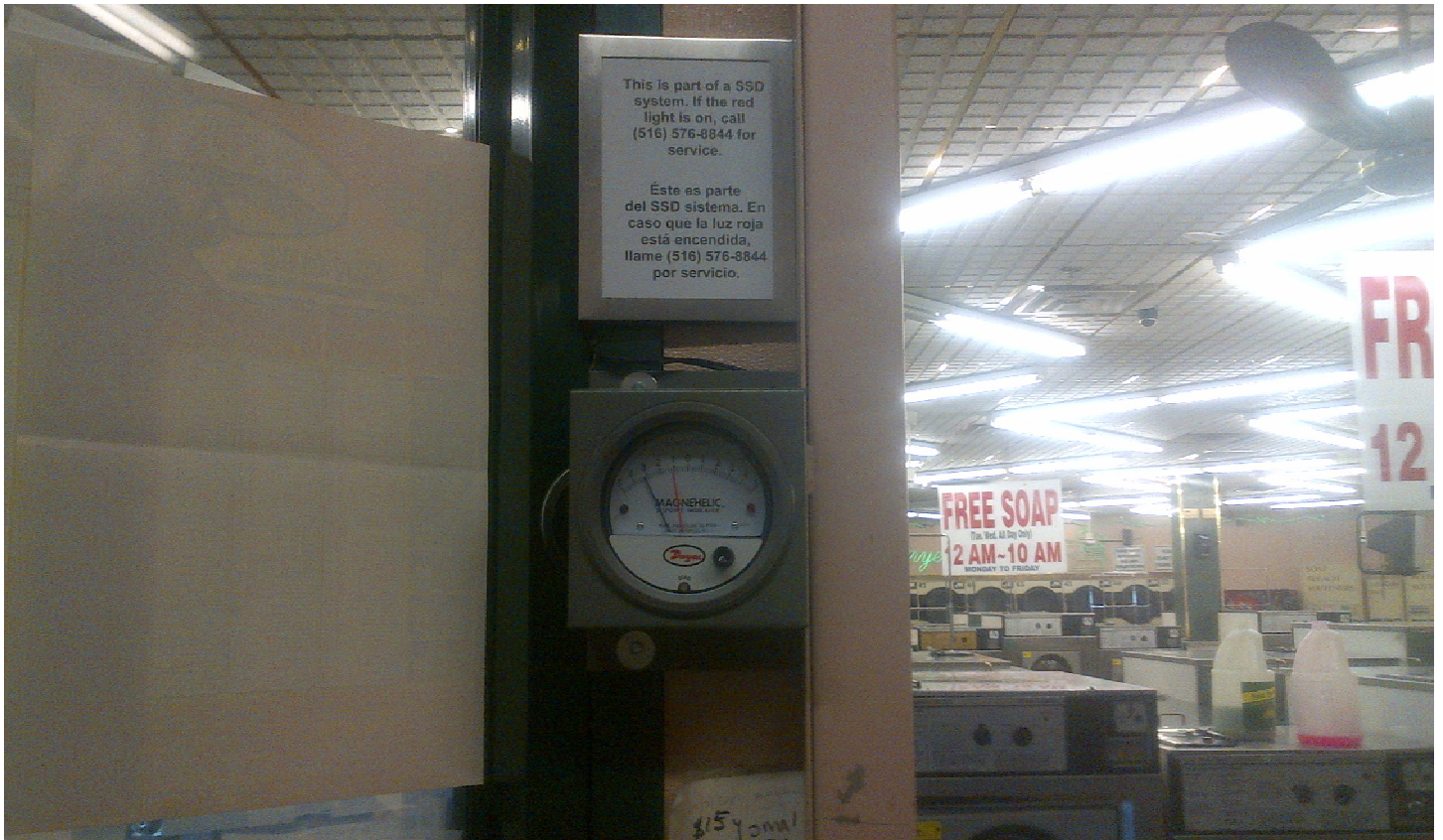
Vacuum gauge with indicator light
