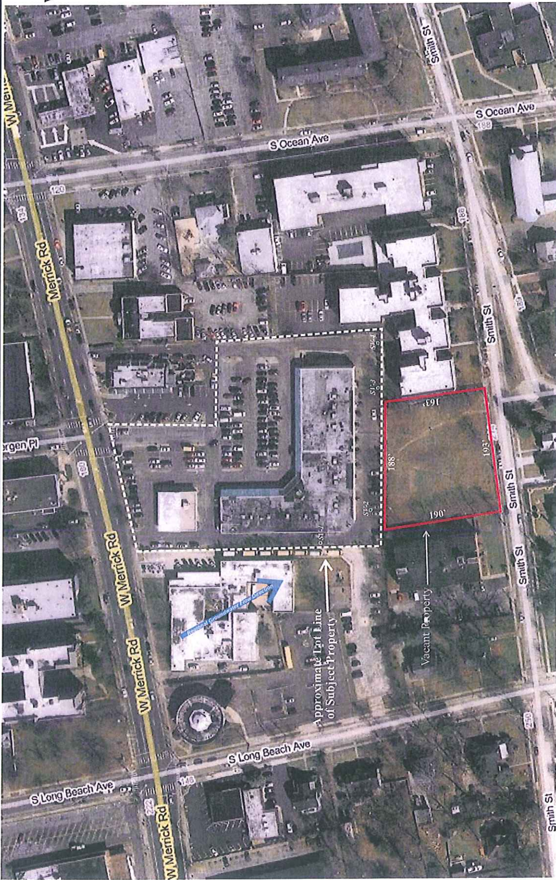
Figure 7- Aerial Photograph of Elks Plaza and Surrounding Properties
