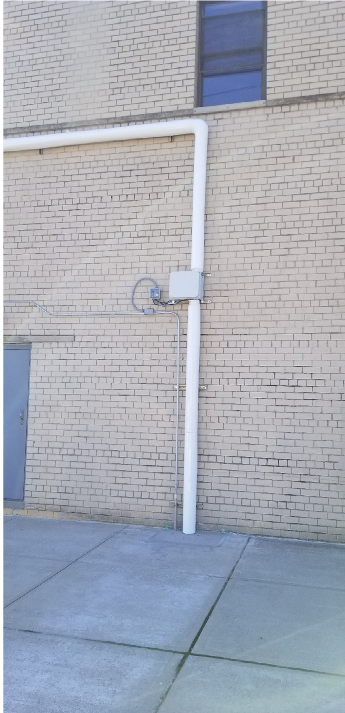
SSDS-2 - View of exterior piping for SSDS riser
