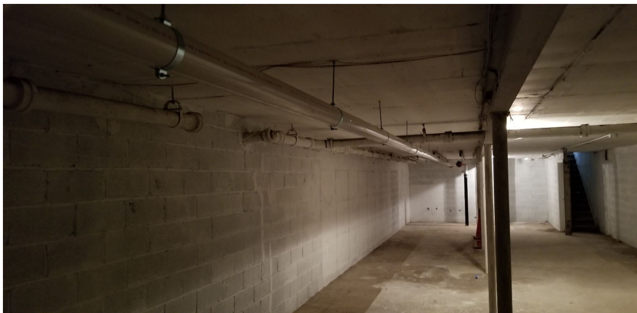
SSDS-14 - View of interior SSDS piping
