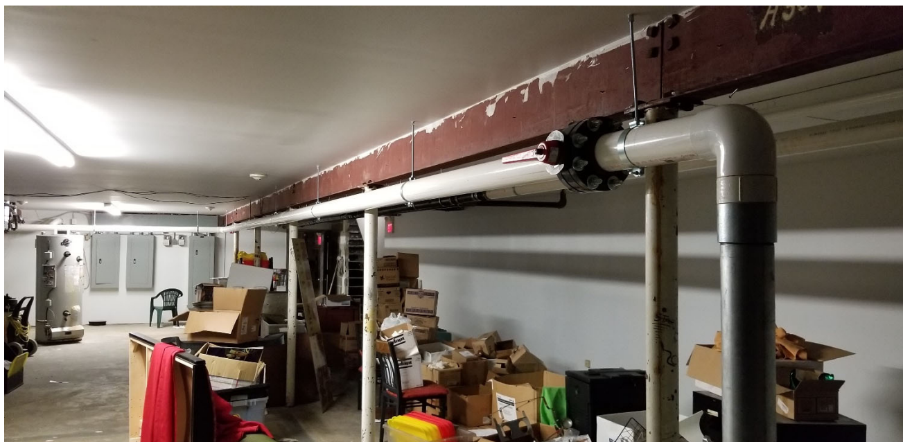
SSDS-6 - View of interior SSDS piping
