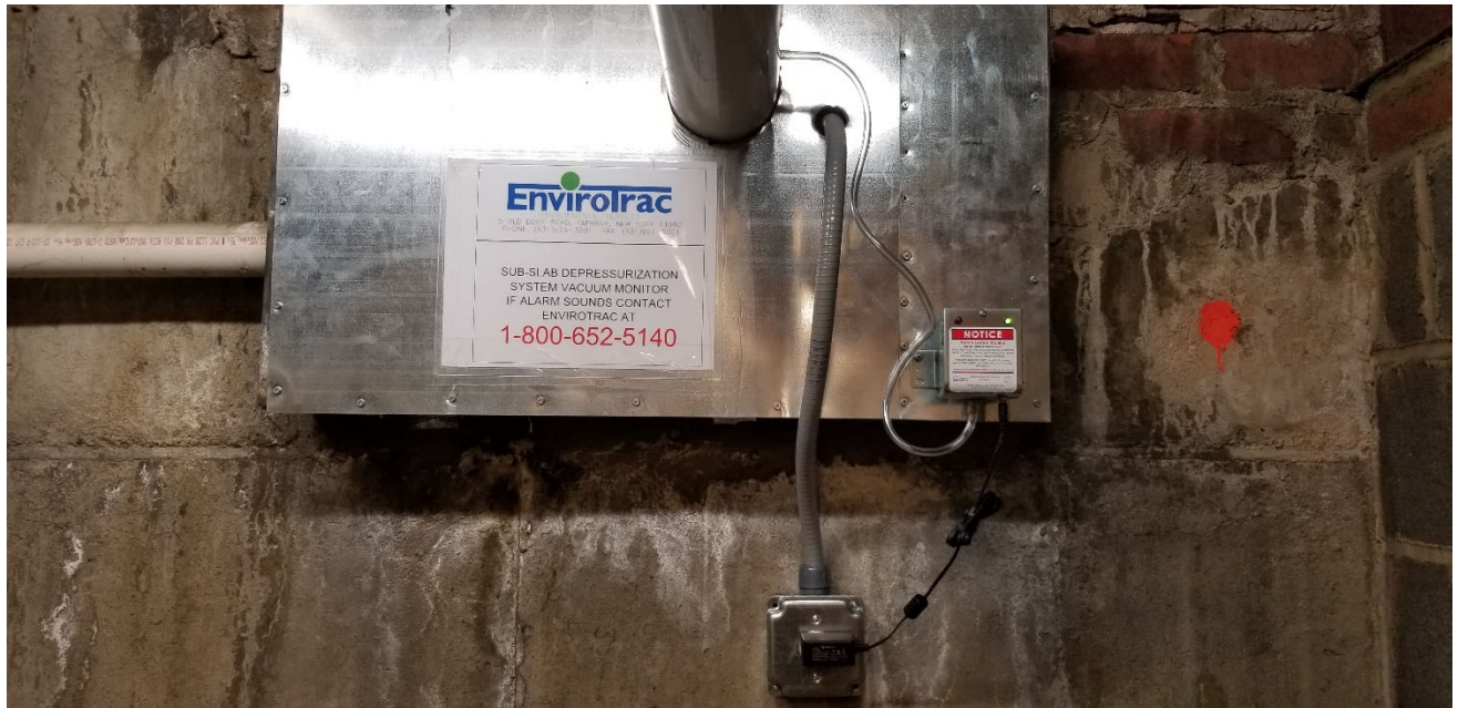
SSDS-3 - View of SSDS Alarm
