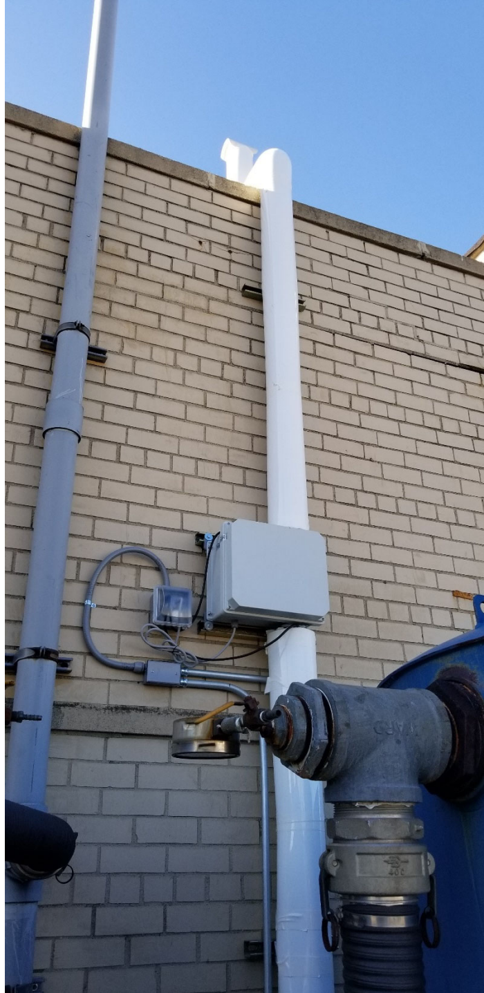
SSDS-1 - View of exterior piping for SSDS riser
