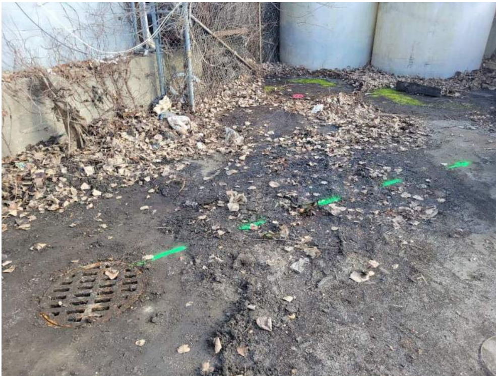
Photograph #4 Date: 01/18/2022 Description: Utility markout.
