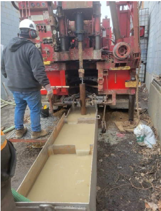
Photograph #7 Date: 01/19/2022 Description: Drilling at GEO-01.
