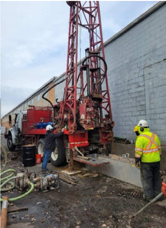
Photograph #5 Date: 01/19/2022 Description: Drill rig setup at GEO-01.
