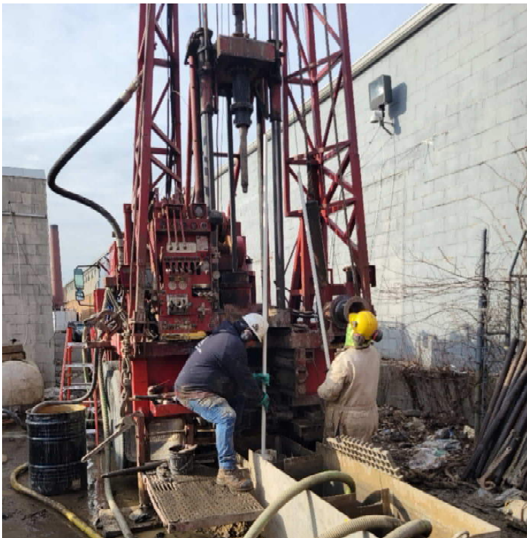
Photograph #44 Date: 01/25/2022 Description: Grouting GEO-02.
