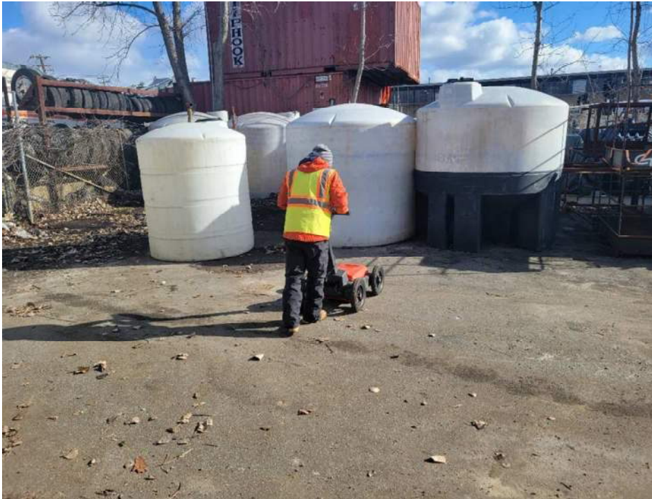
Photograph #3 Date: 01/18/2022 Description: GPR investigation.
