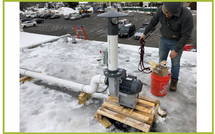
Photo #8: Installation of blower on roof.
