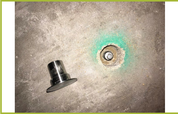
Photo #7: Typical vapor monitoring point (Vapor Pin)
