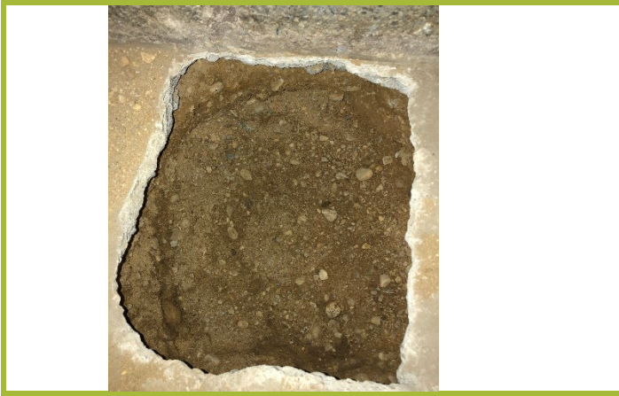
Photo #1: Typical Extraction pit prior to installation of riser.
