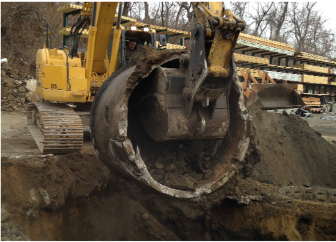
Removal of the cesspool.
