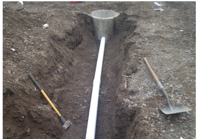
View of completed exterior trenching.
