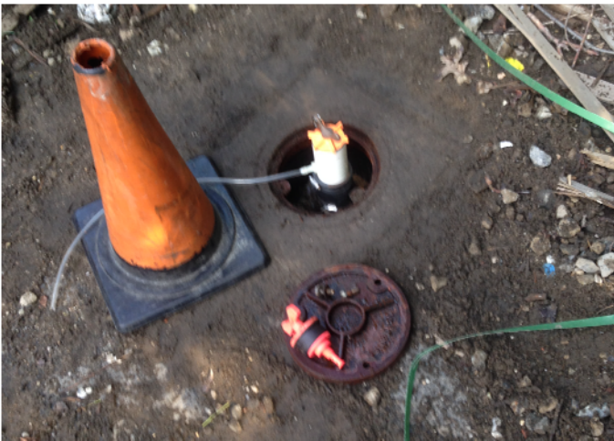
Existing groundwater monitoring well capped for pilot test.
