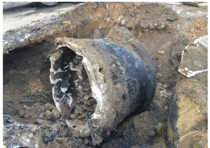
View of cesspool.
