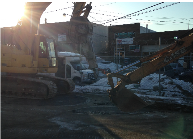
View of breaking up the asphalt.
