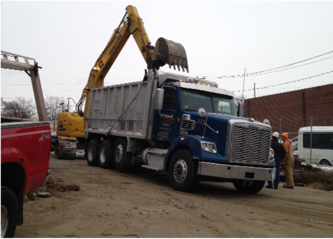
View of trucking out soil.
