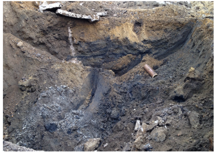
View of the excavation.
