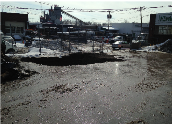
View of the excavation.
