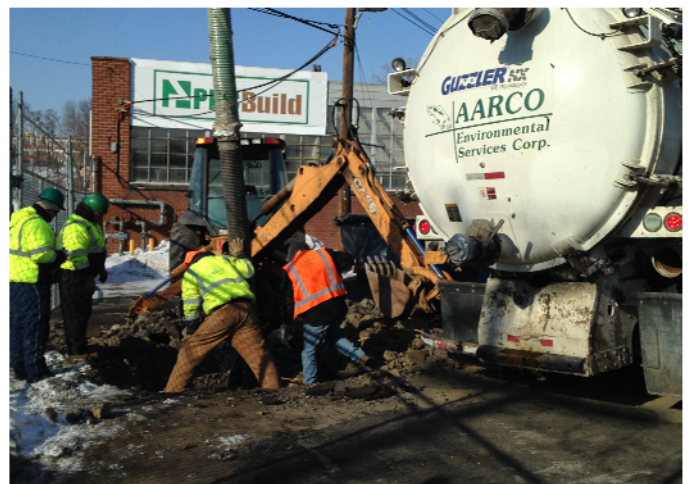
View of guzzler and excavator removing material from cesspools.
