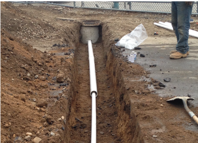
View of 2-inch pipe inside 4-inch pipe (casing).
