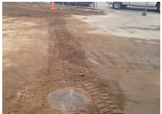
Backfilled trench for exterior piping.
