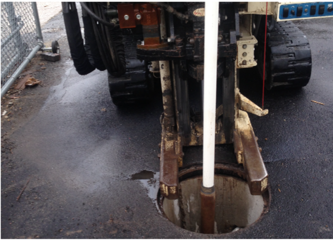
Installation of exterior SVE well.
