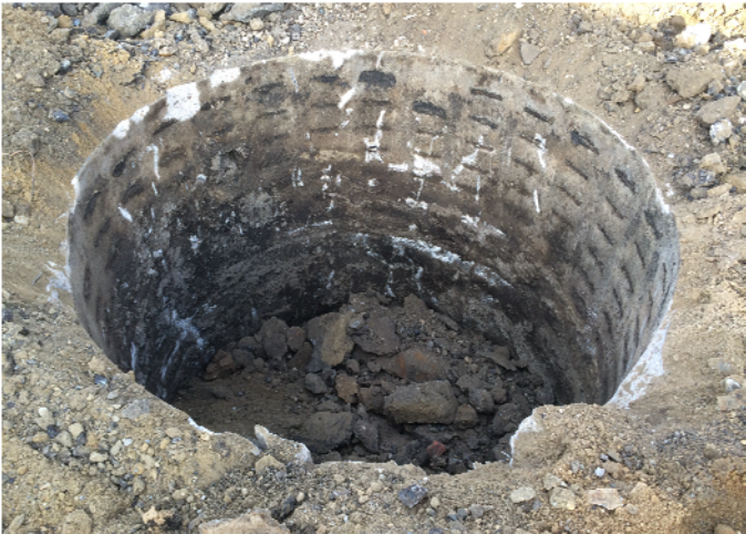
Interior view of cesspool.
