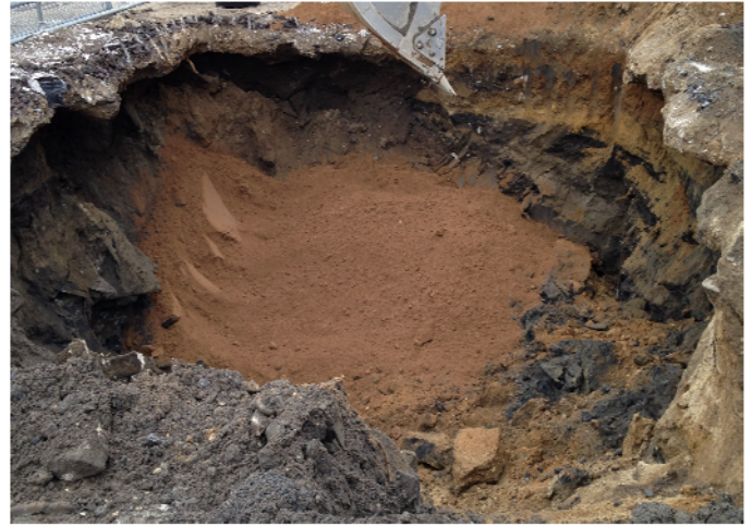
View of backfilling.
