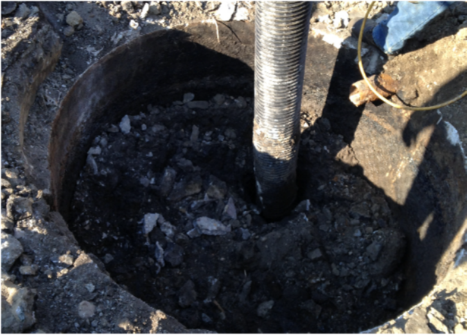
View of guzzler removing material from the cesspool.
