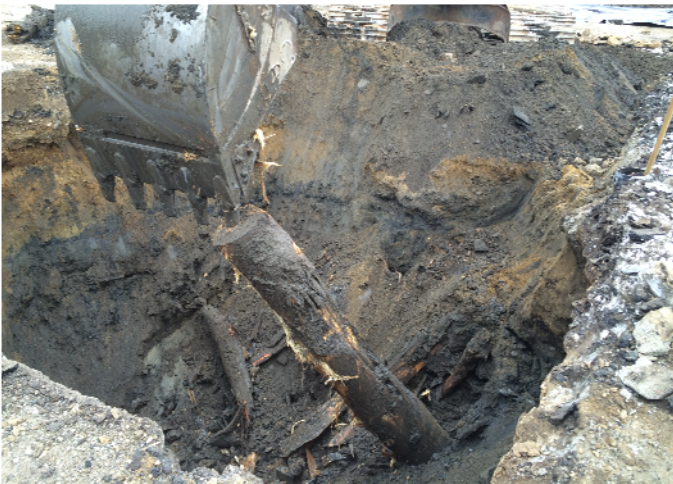
View of debris encountered within excavation.
