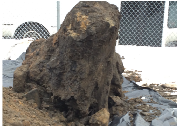
View of debris encountered within excavation.
