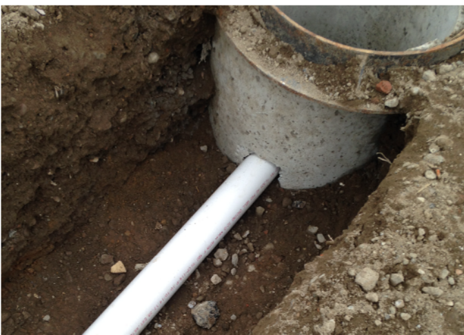
View of exterior piping entering 23-inch manhole.
