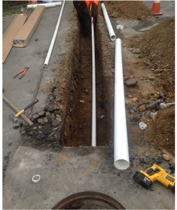
View of exterior trenching.
