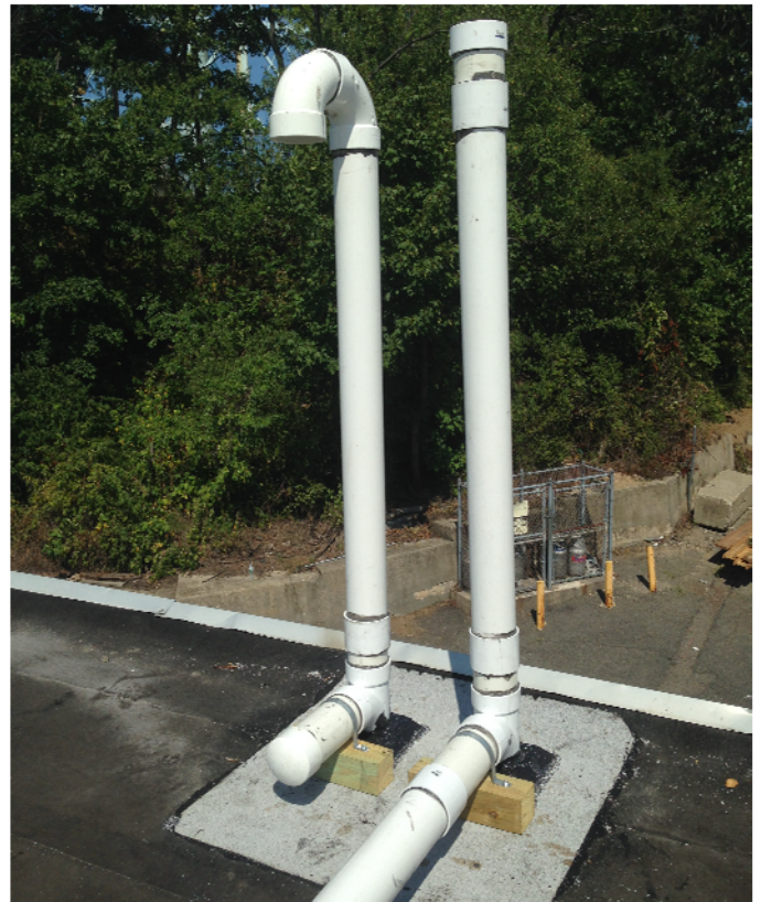
View of roof riser.
