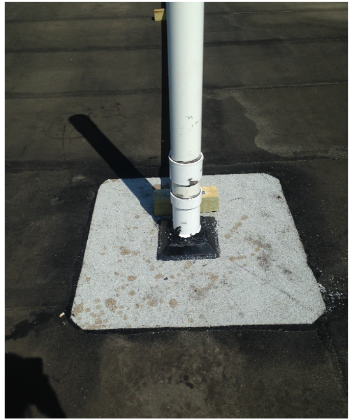
View of pitch pocket for roof riser.
