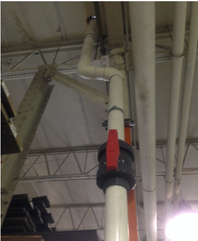
View of interior duct.
