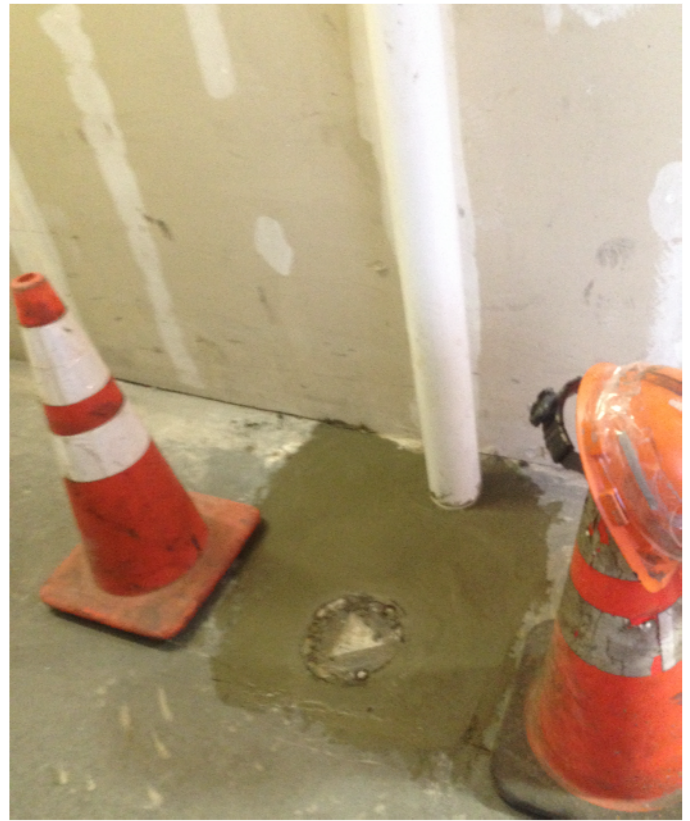
View of completed SSD-4 trenching.
