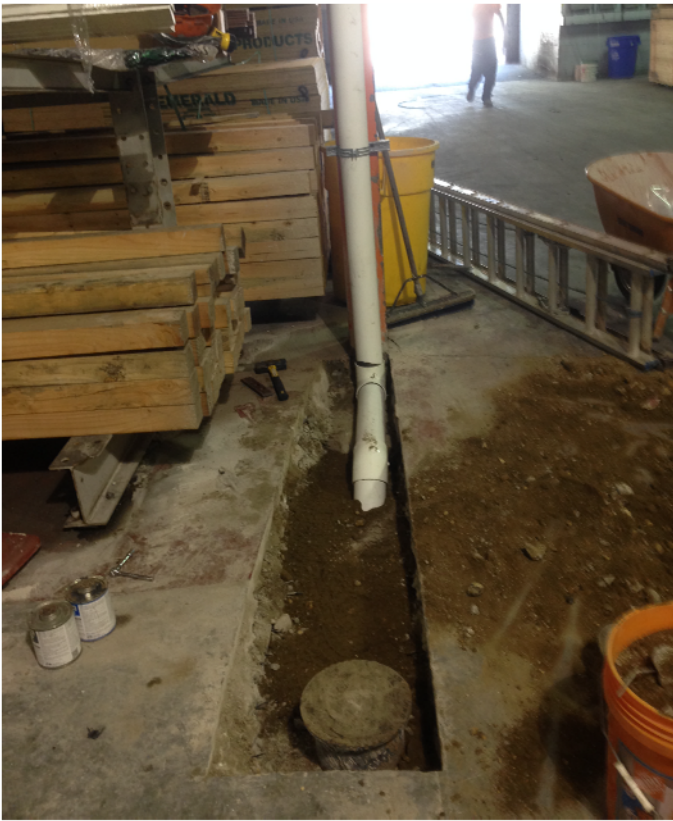
View of SSD-5 trenching.
