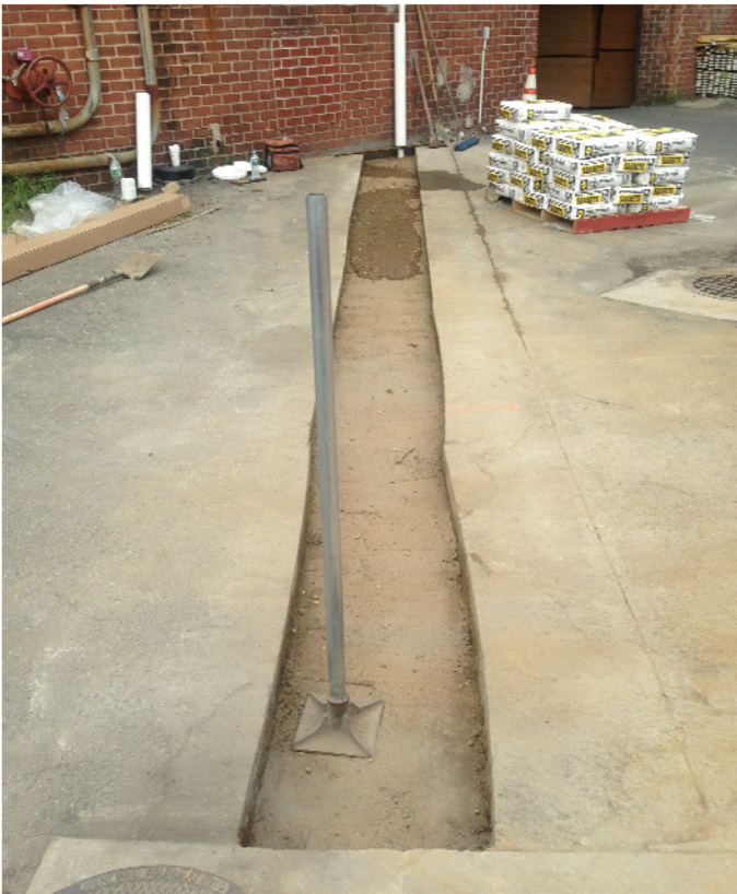
View of exterior trenching.
