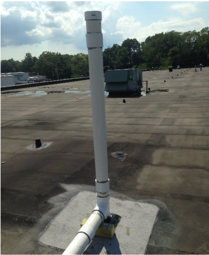
View of roof riser.
