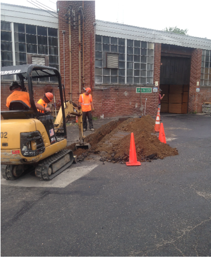
View of exterior trenching.
