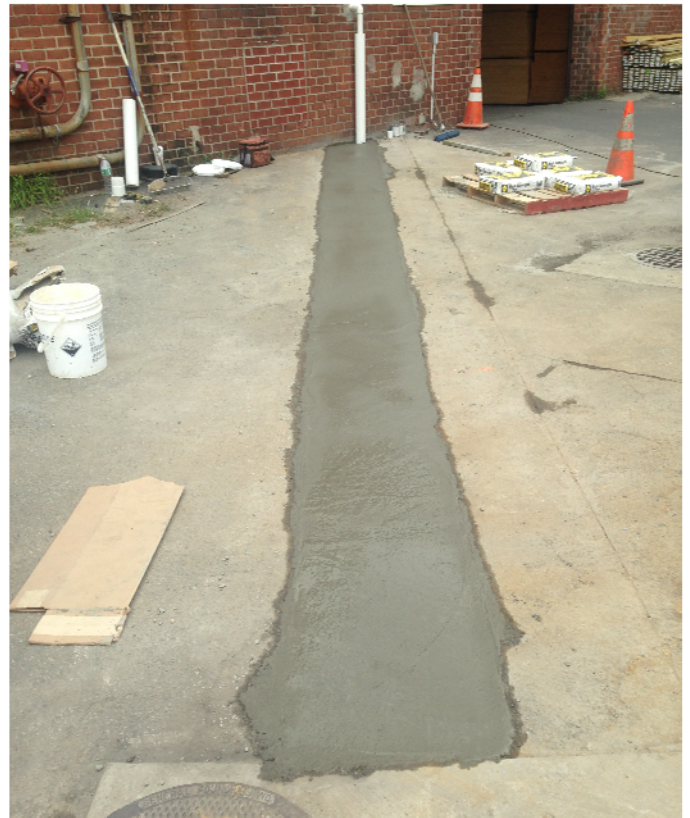
View of completed exterior trenching.
