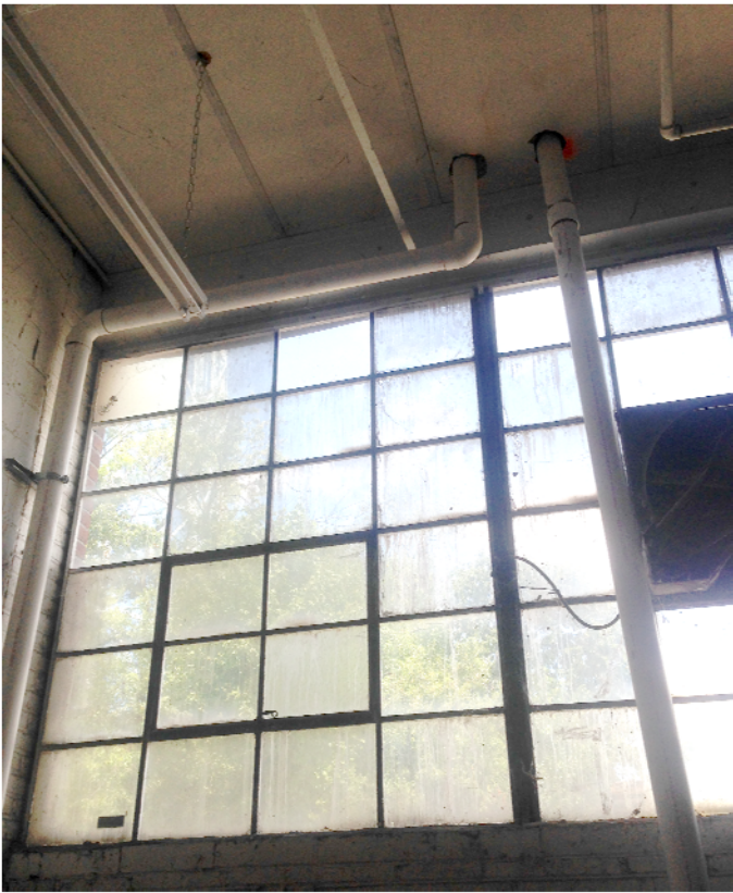
View of interior ducts.
