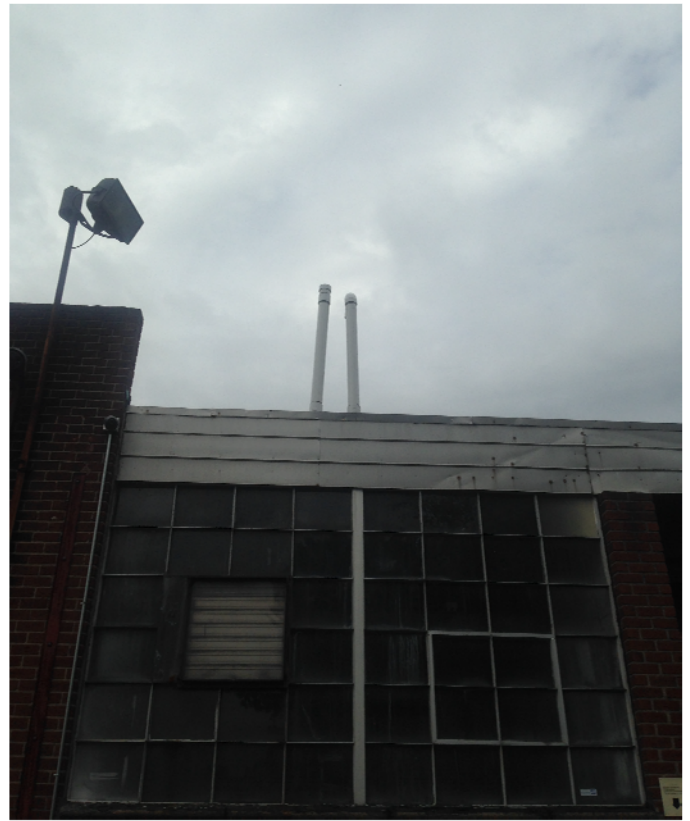
View of exterior risers.
