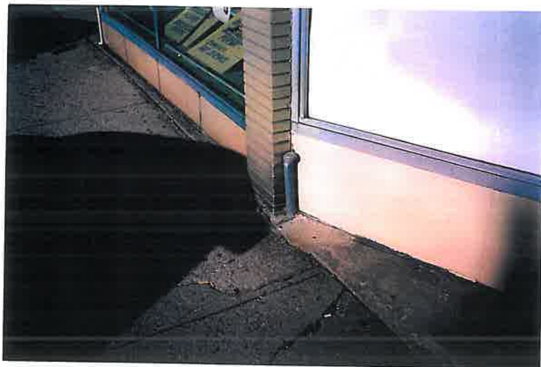
Photo 6. UST Vent Line in Front of Dry Cleaners.
