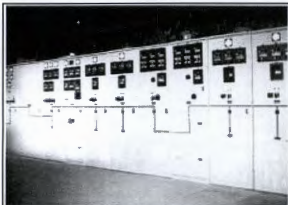
13.2kV Metal-Clad Switchgear for Large Oxygen Plant
