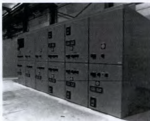
15kV 500MVA Indoor Line-Up
