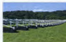
Place supports, attach rails, then level rail supports quickly prior to pouring concrete
