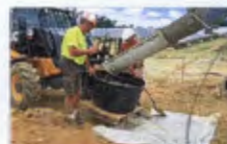
Gen4 Pour-in-Place™ Ballasted Ground System with round forms shipping Q4 2015: less concrete, faster install, steeper slope
