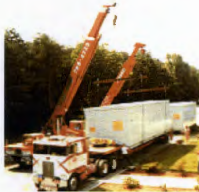
Climatized 13.8kV Metal-Clad for Petrochemical Plant
