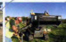
Pouring bucket on bobcat for concrete pouring of Pour-in-Place™ forms on sensitive landfill caps
