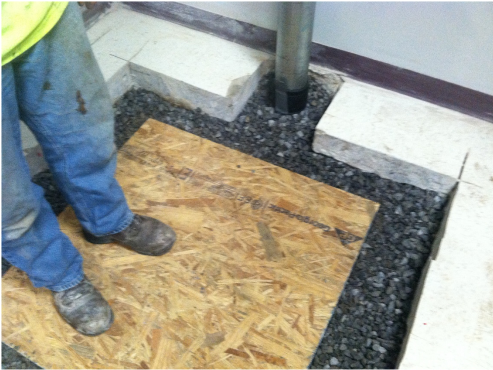
Riser Pipe Installed and Surrounding Space Filled with Stone.
