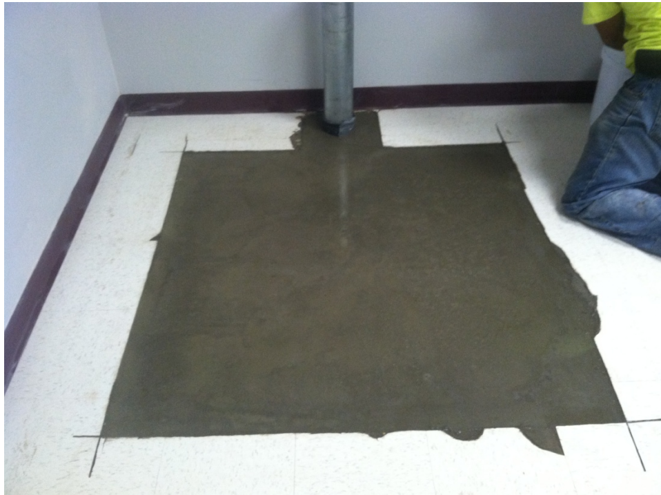
New Floor Slab
