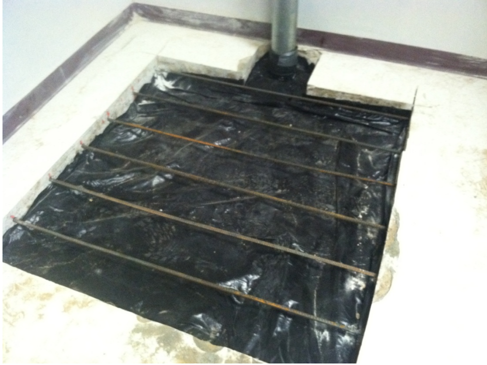
Plastic Sheetting to Contain Concrete. Re-bar.
