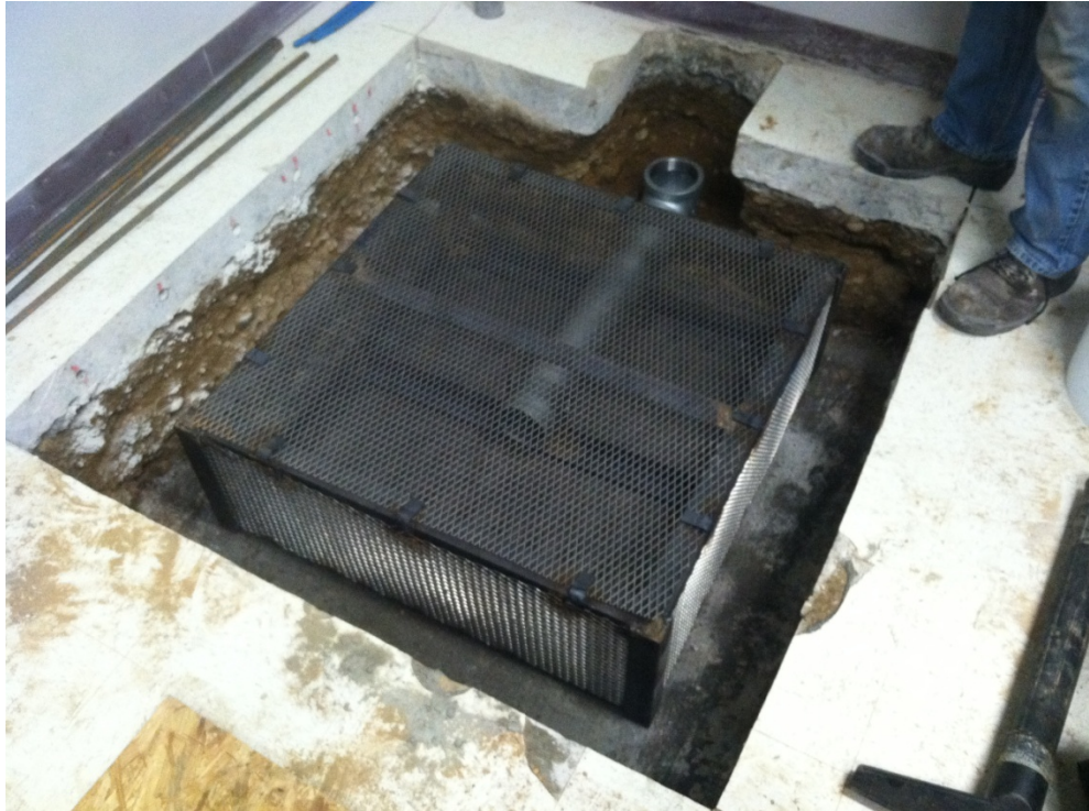
SSVM Suction Pit with expanded steel cage
