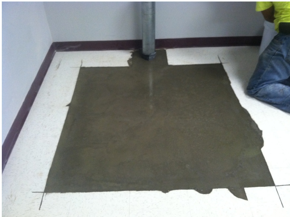
SSVM suction pit with new floor
