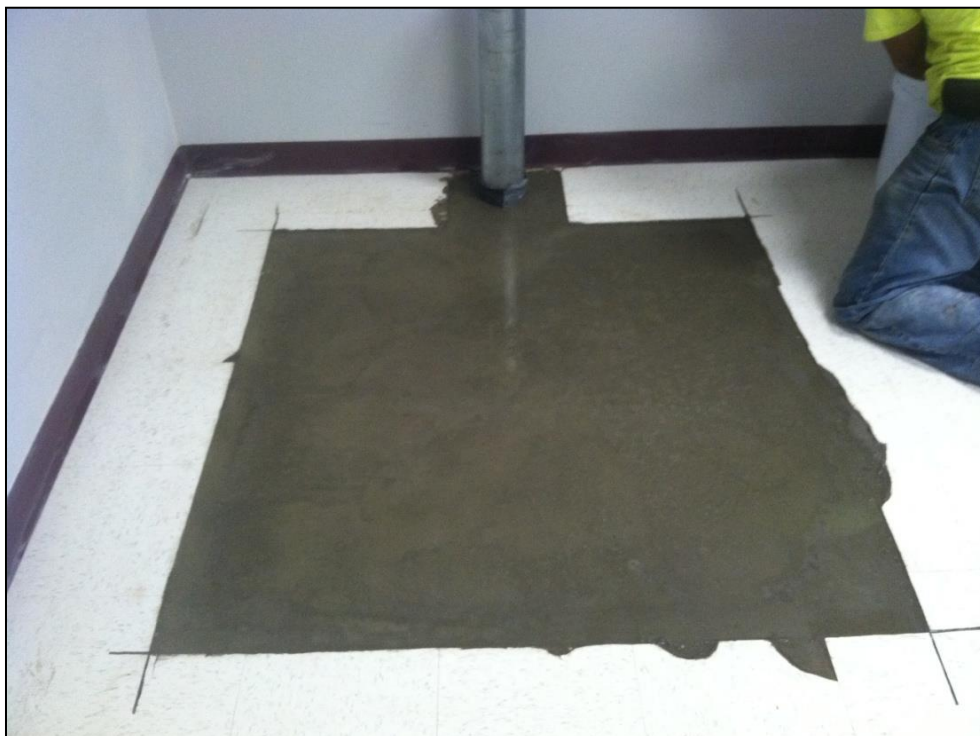
SSVM Suction Pit with New Floor
