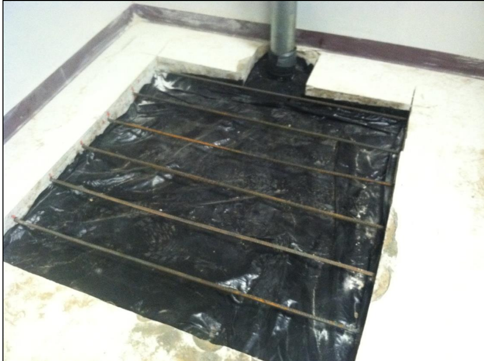
SSVM Suction Pit with Vapor Barrier and Rebar
