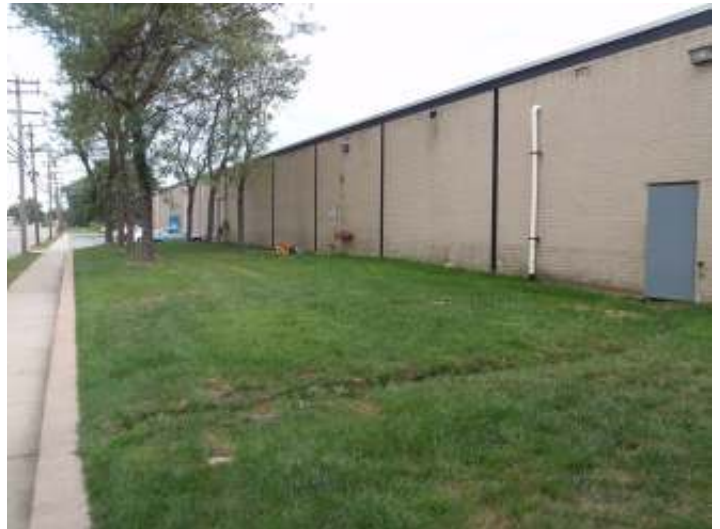
AOC—4: Cutting Oil Release Area. Looking east.
