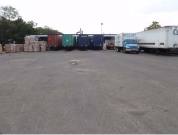
AOC—1: Former Seepage Lagoon Area. Looking west.
