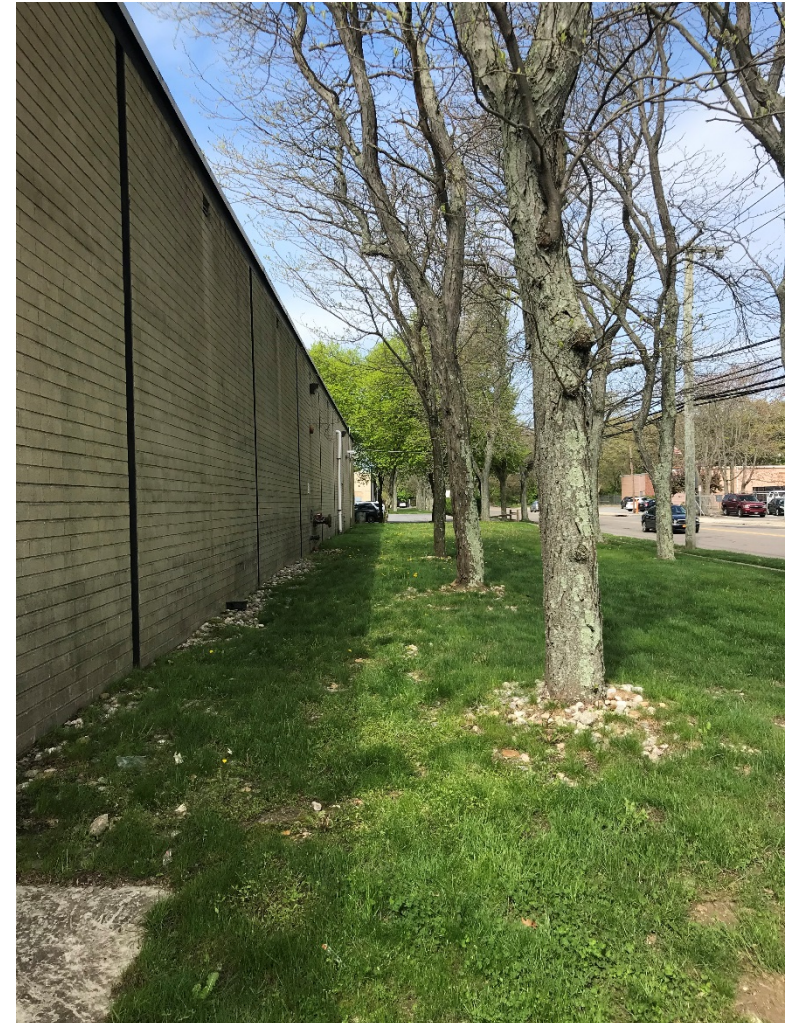
Photo 4: (5-6-2019) AOC 4. Exterior portion of AOC 4. On north side of Site building. Looking west.
