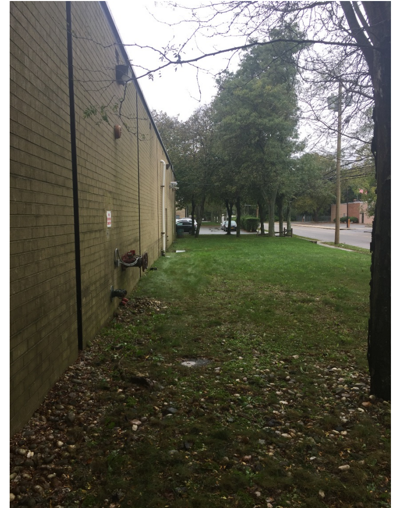
Photo 4: (10-15-2018) AOC 4. Exterior portion of AOC 4. On north side of Site building. Looking west.
