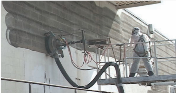
Hydro-blasting technique will contain asbestos and lead paint as it's removed
