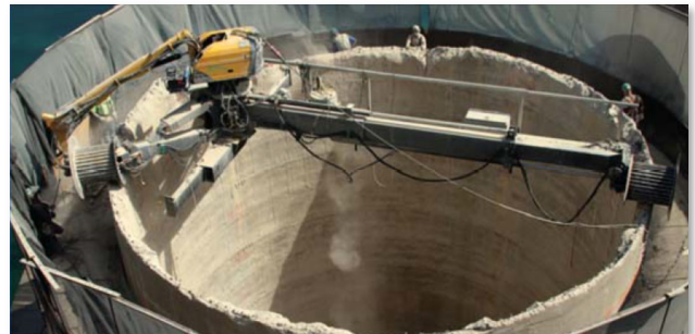
MANTIS™ system removing a stack similar to the HFBR Stack
