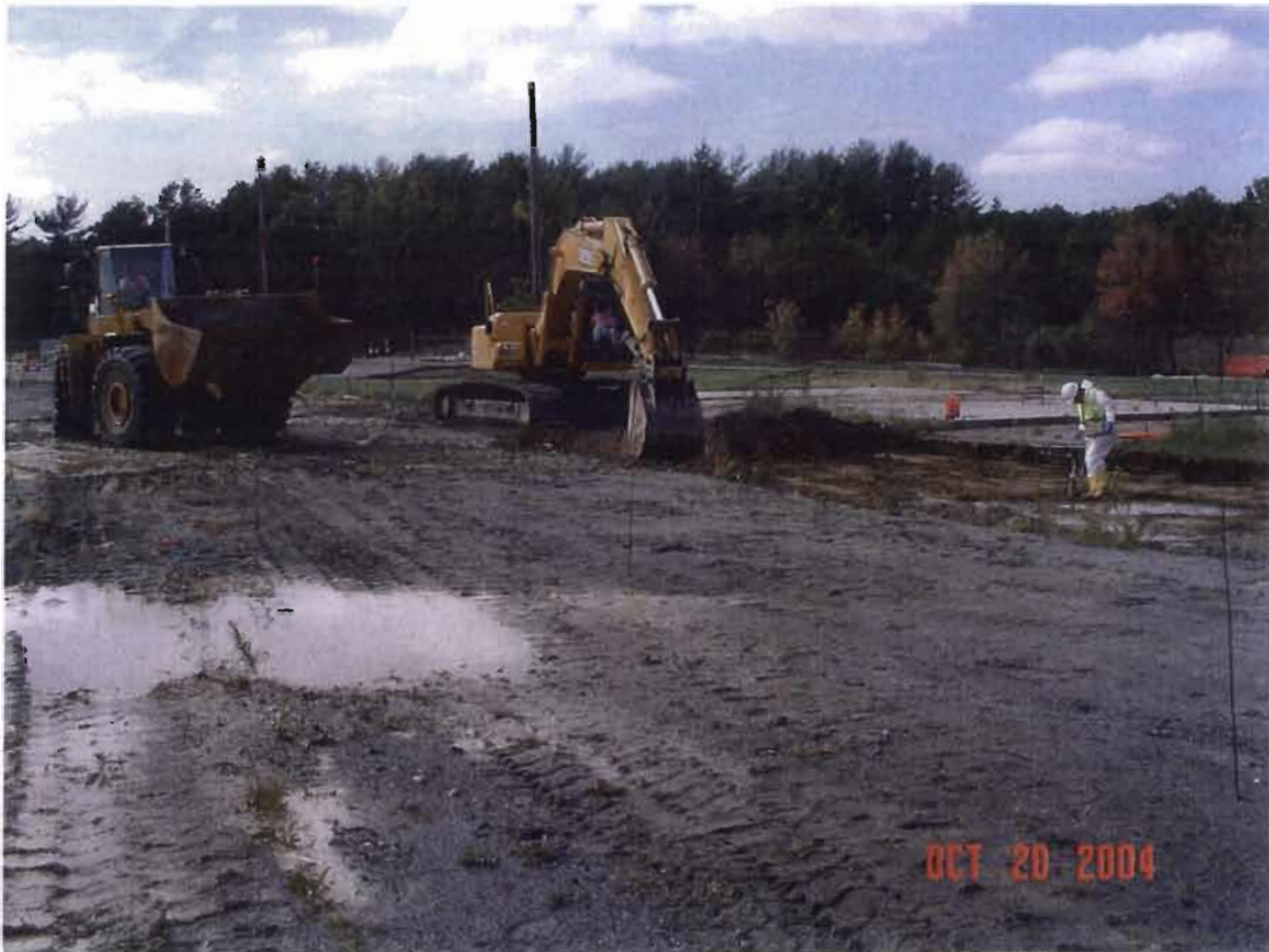
Photograph 2 – Excavating and surveying at the former HWMF.
