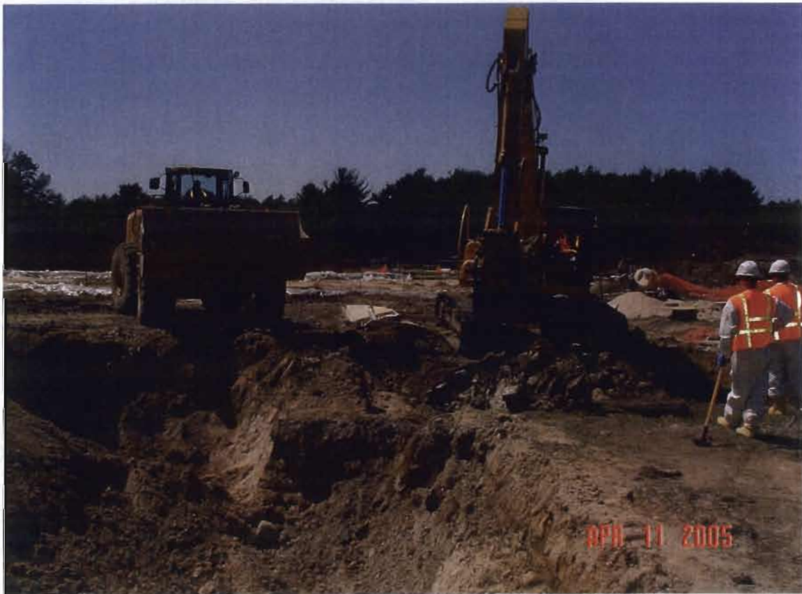
Photograph 3 – Uncovering trench at the former HWMF.
