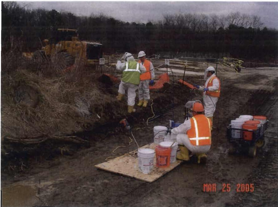
Photograph 4 – Applying fixative to slant-holes at the former HWMF.
