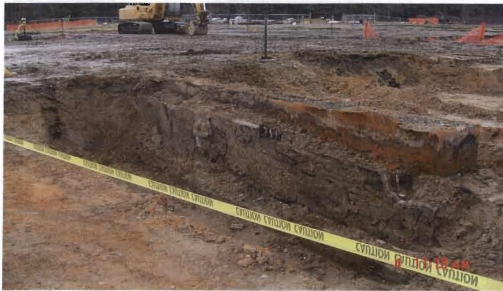
Photograph 6 – Discovered sub-surface structure as the former HWMF.
