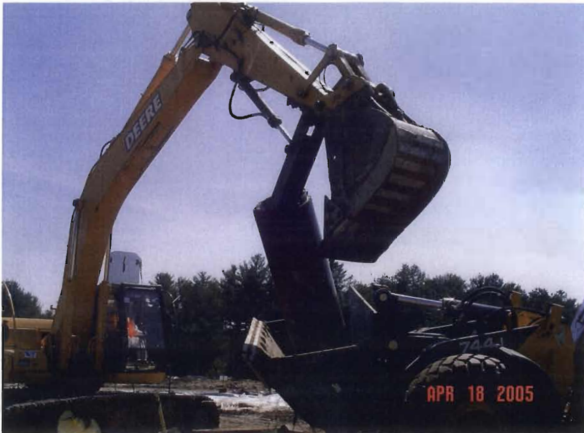
Photograph 5 – Removal of vertical hole at the former HWMF.
