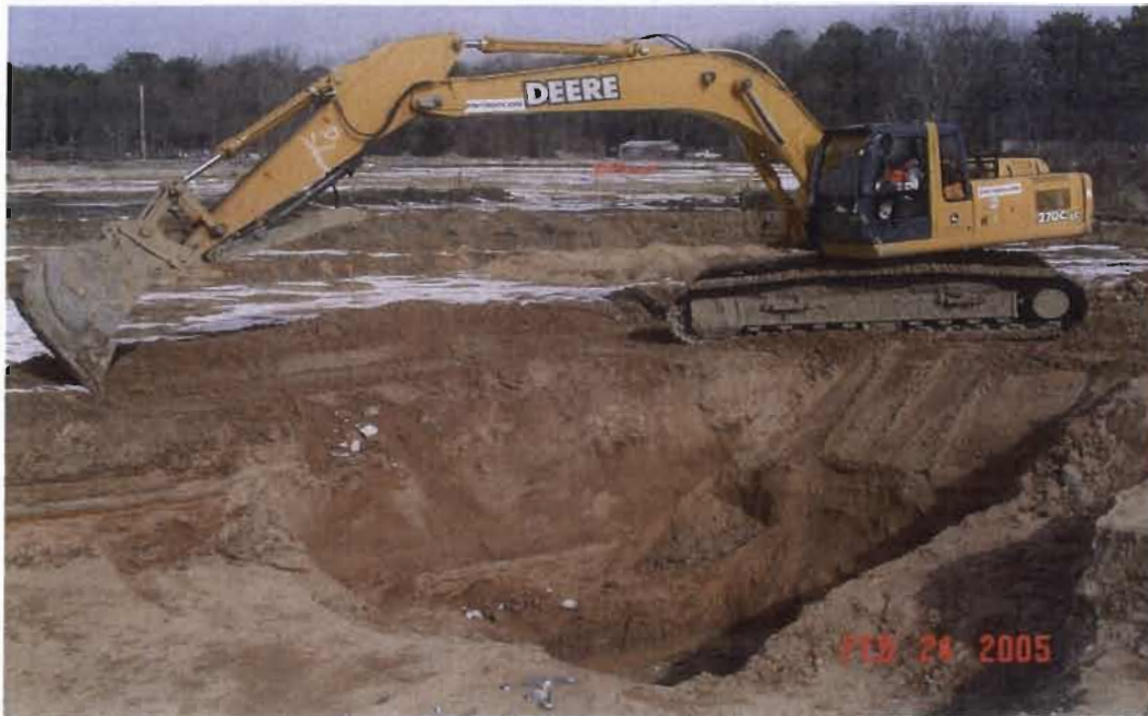
Photograph 1 – Soil removal at the former HWMF.
