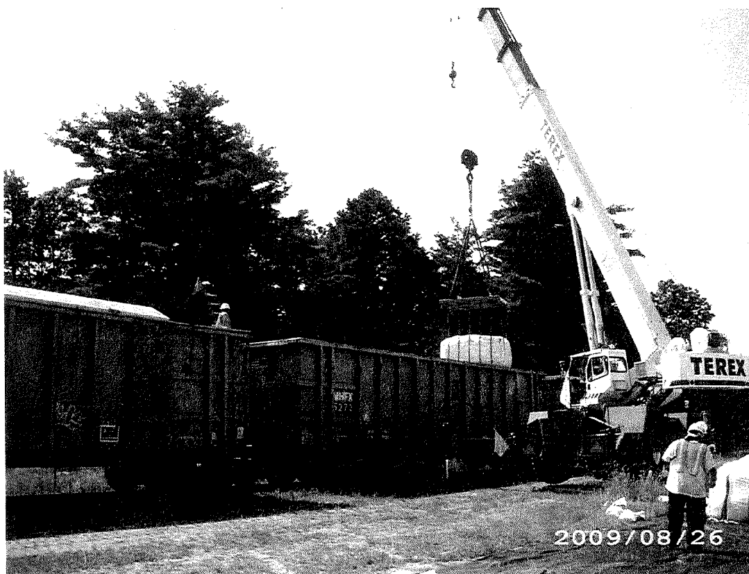
Photograph 3 – Loading Lift Liner containing contaminated soil into railcar at the WLA.
