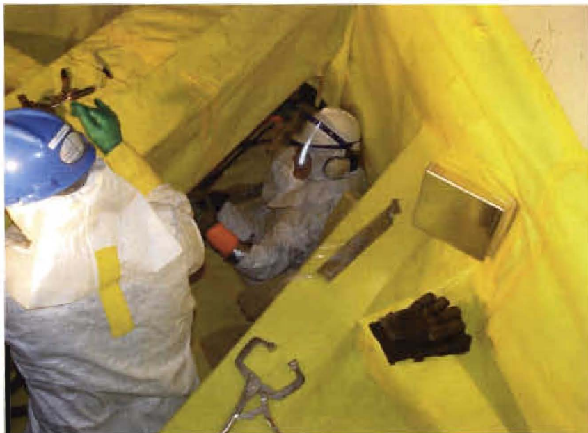
Photo 1 Control Rod Cutting and Removal
