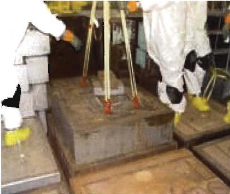
Photo 3 Roof Plug Removal
