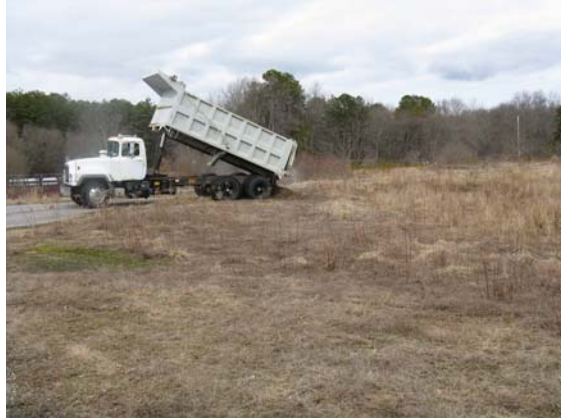
3/2/10 – Excavated landscape soil transferred to former hazardous waste management facility for use as fill
