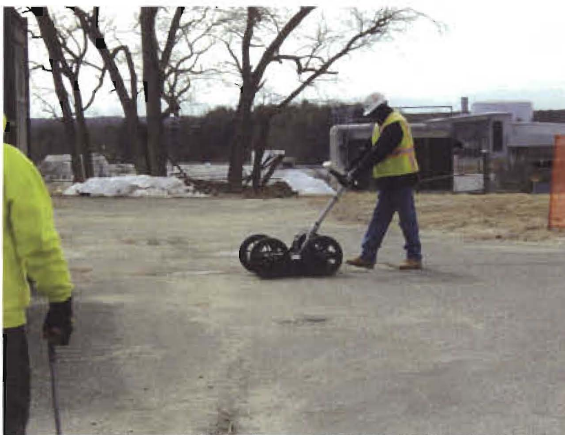
Photograph 1 – Marking out utilities with ground-penetrating radar prior to excavation
