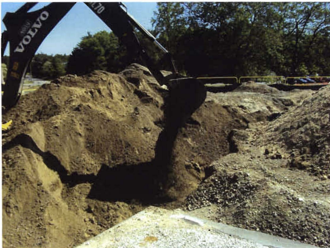
Photograph 8 – Backfilling Phase II Trench
