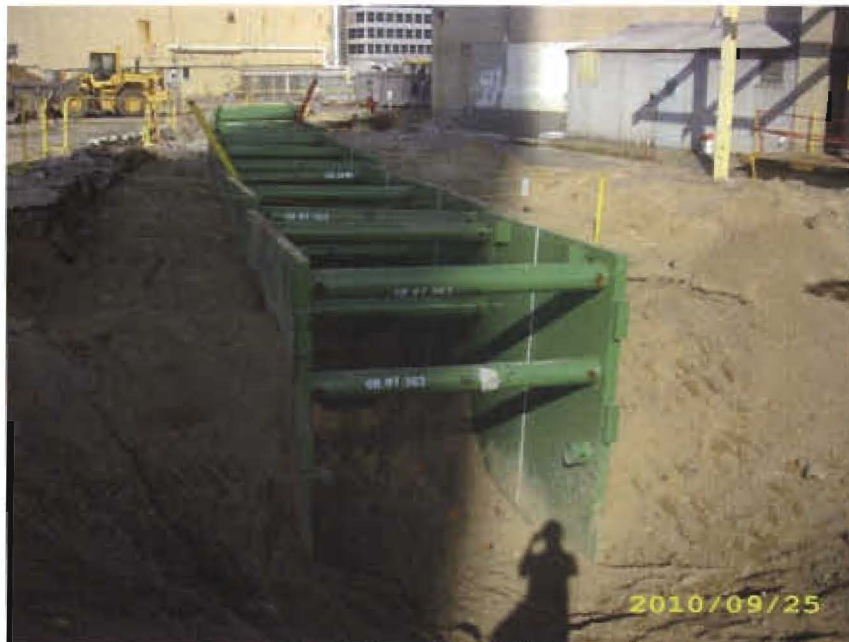
Photograph 4 – Trench boxes installed in Phase III, Trench 4
