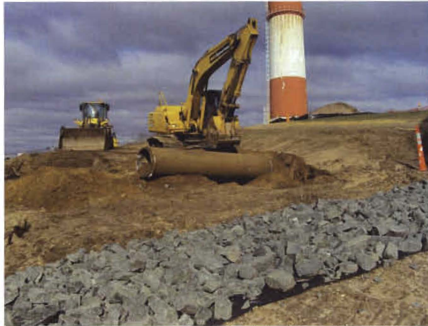
Photograph 2 – Removal of 30-inch duct during Phase I of the project
