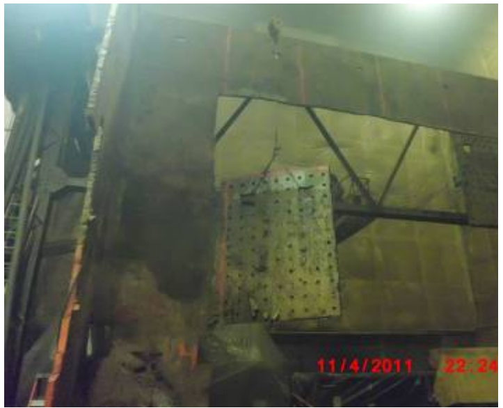
A large section of the north outer wall plate being lifted.
