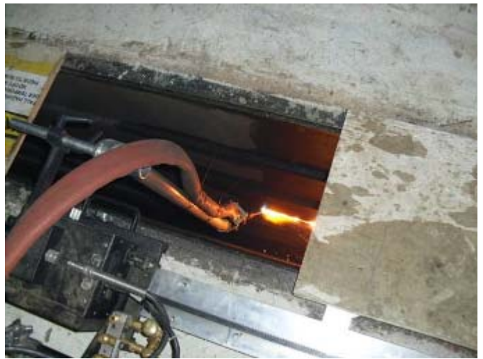
View looking down through scanner slot. Bug-O® drive can be seen in foreground. The oxy-propylene torch can be seen in the background.
