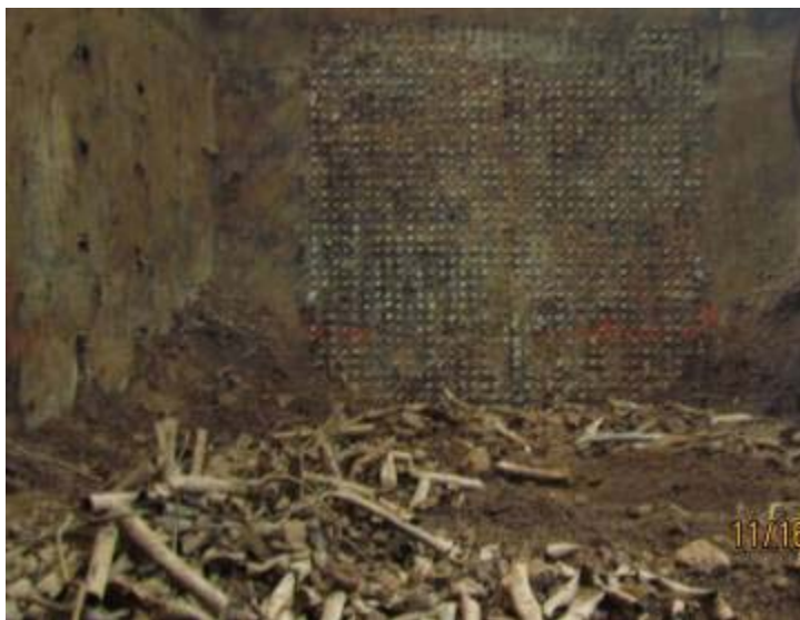
View of the inner biological shield looking south from the north wall opening. At this time, the majority of the wall concrete has been demolished; the concrete and the experimental port tubes can be seen on the floor.
