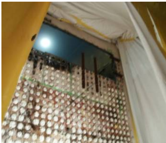
South outer biological shield wall after removal of the upper section. Note the two horizontal and vertical retaining bars which prevented the cut steel plates from falling outward during removal.
