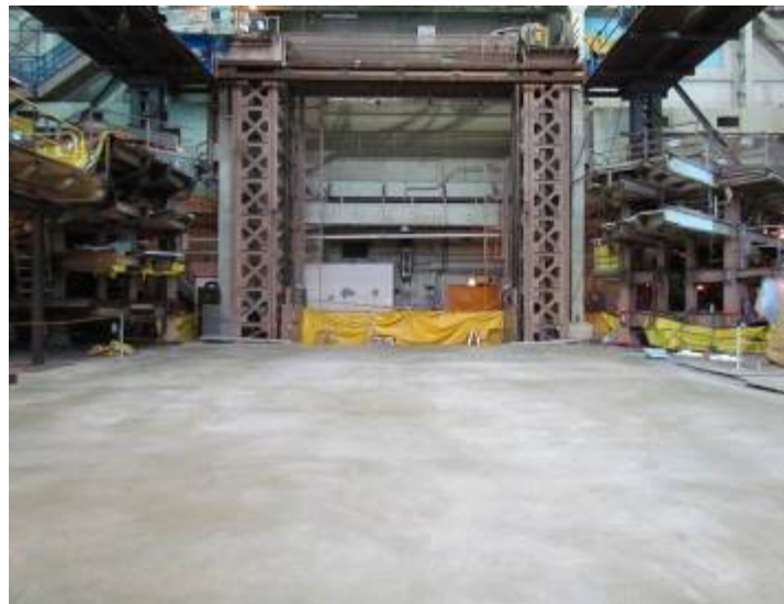
View of the Building 701 high bay looking south where the reactor once stood. The charging elevator can be seen in the background.
