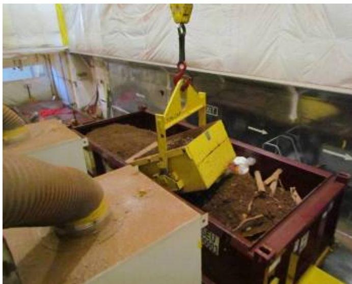
A view of the self-tipping 8-ton hopper that was used to load the majority of the concrete rubble into the waste intermodal containers.
