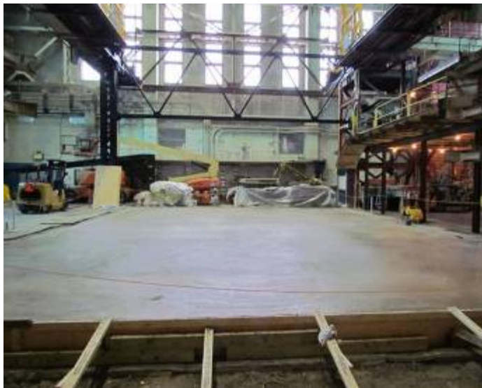
View of the biological shield footprint looking north after placement of the final cap.
