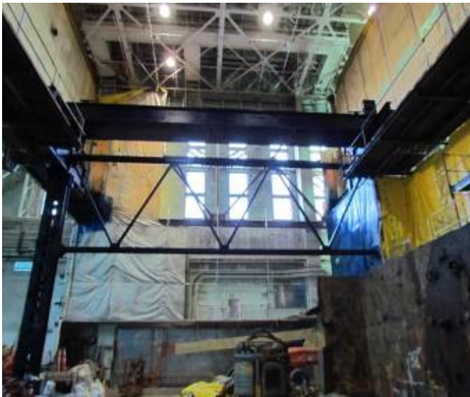
Removal of the CCE in progress viewed from the south at floor level. In this photo the majority of the north and west fabric walls have been removed.
