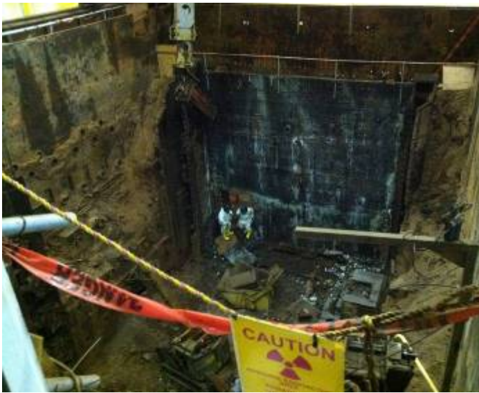
August 21, 2011 – First entry of personnel into the biological shield interior since original construction in the late 1940s.
