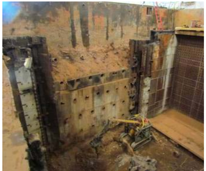
View of the Brokk remote manipulator fitted with a clamshell bucket loading concrete from the east wall.
