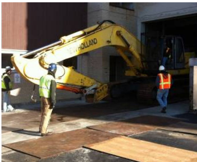
New Holland excavator being brought out of Building 701 after completion of its use on the project.
