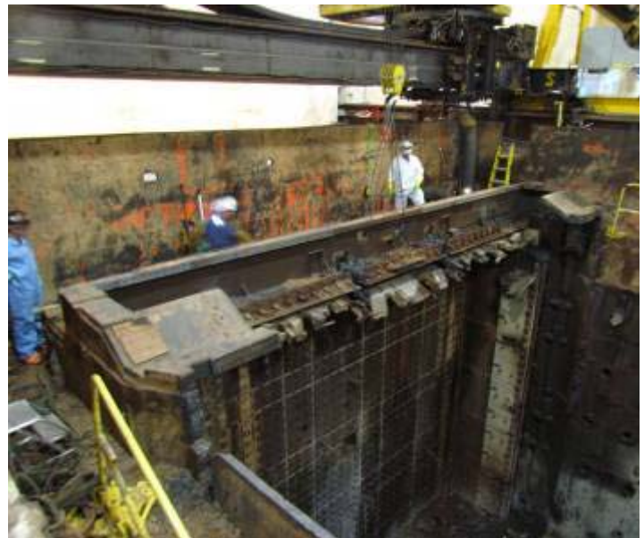
View with roof removed at north wall
