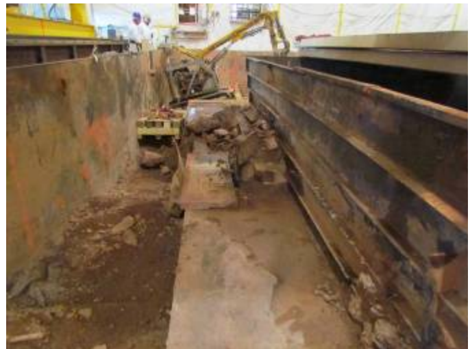
The Brokk remote manipulator fitted with a hydraulic breaker hammer being used to break the roof concrete. The Brokk manipulator was used extensively throughout the project when the larger Gradall and New Holland excavators were not effective.
