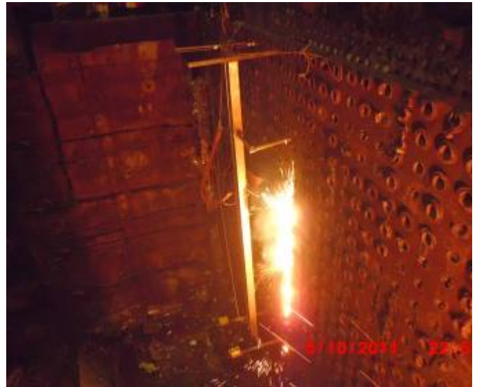
Bug-O® track installed on a BSA-designed vertical rack with magnetic securing devices. This method was extensively used to cut the inner biological shield walls.
