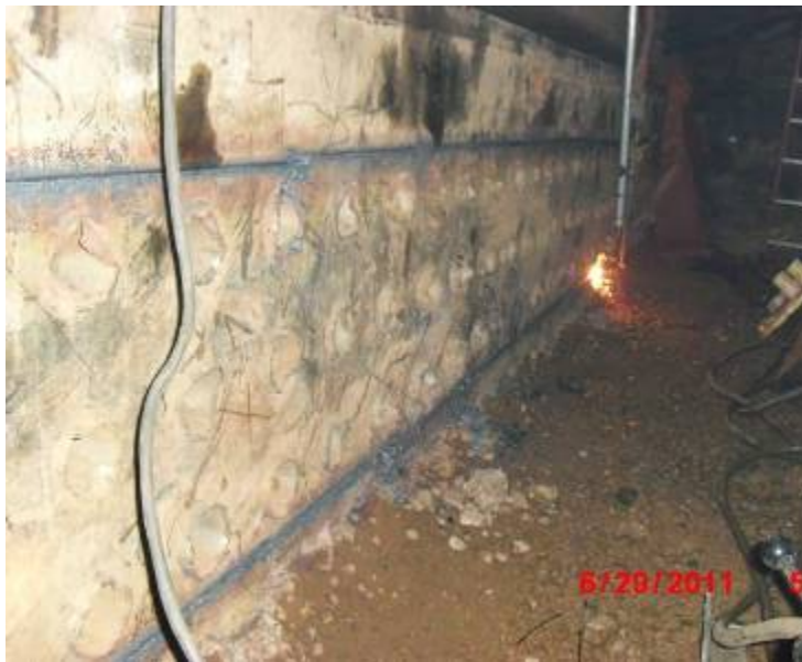
One of the tools designed and fabricated by the BSA team. This is an oxy-propylene torch on a 20+ foot long extension rod. At the top of this rod is the Bug-O® drive which controlled the horizontal movement of the torch.
