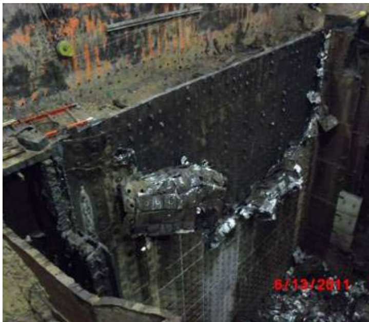
View of the north inner wall showing the 4-inch thick aluminum and steel thermal shield. This shield, which surrounded the walls of the outlet air plenums had to be removed to access the inner wall plates for cutting.
