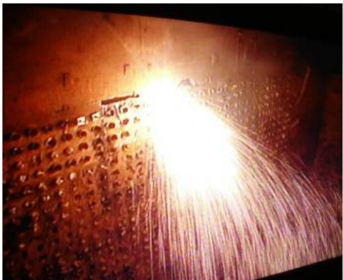
South outer wall cutting from the inside by remote camera.
