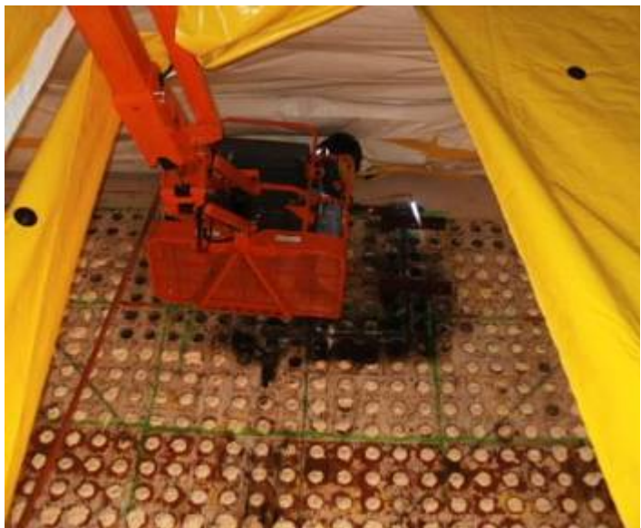
BSA technician using a hand-held torch to cut the contaminated section of the south outer biological shield wall.
