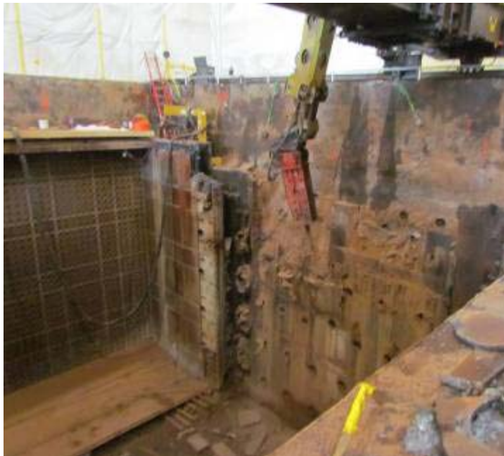
View of the Gradall excavator fitted with the hydraulic breaker hammer breaking west wall concrete.
