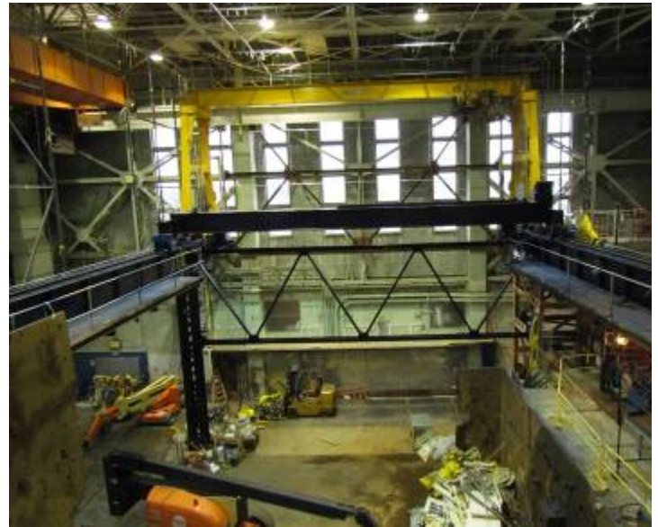
View of the high bay from the south at elevation 140'. In this photo, all of the CCE fabric and side wall framing has been removed. The roof framing can be seen at the top of the photo.
