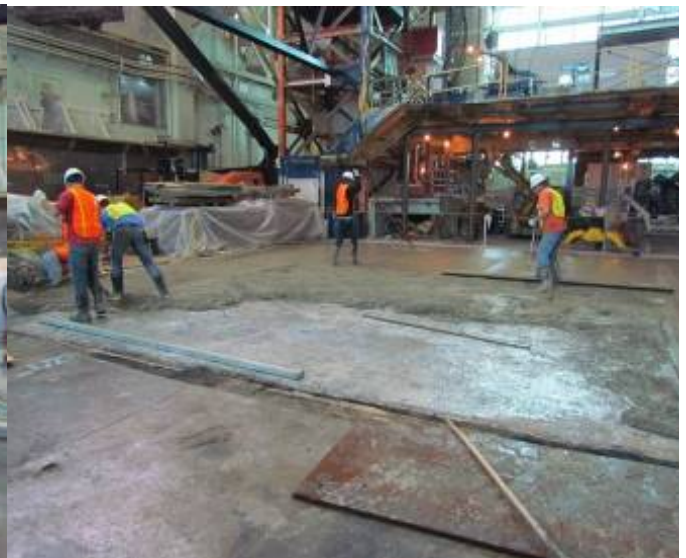
Subcontractor placing final finished concrete cap over the biological shield footprint.
