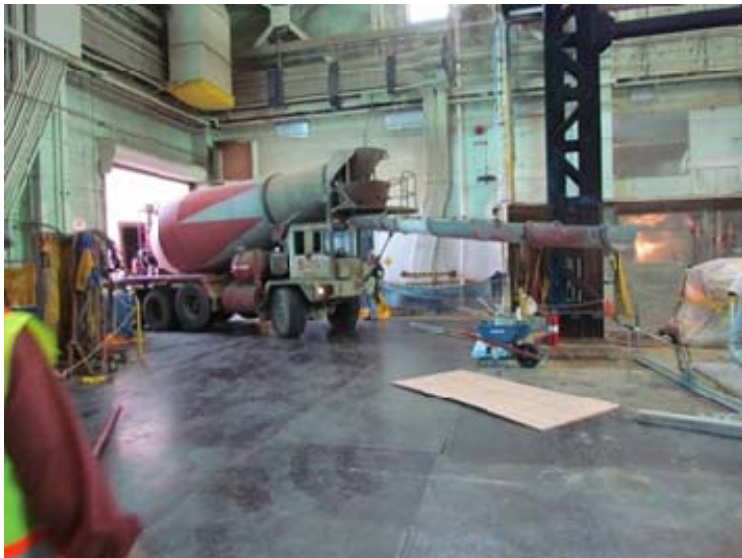
Concrete delivery to place the final cap over the biological shield footprint.
