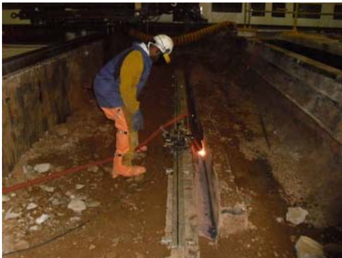
Cutting access hole in roof pan with Bug-O® drive and torch. Access hole will allow insertion of neutron shield cutting tool.
