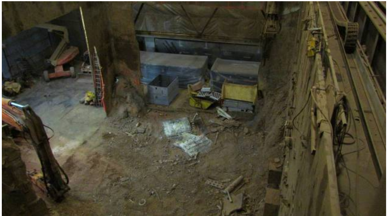
View of the biological shield interior after removal of the majority of the interior concrete and steel wall plates. A small amount of wall concrete can be seen at the lower areas near the floor. The arm of the New Holland excavator can be seen on the left.
