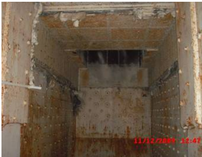
View of the south outlet air plenum from the below ground duct. The opening to the biological shield is the dark square area. This entire area was filled with cementitious grout up to elevation ~109' to support the final reinforced concrete floor over the biological shield footprint.
