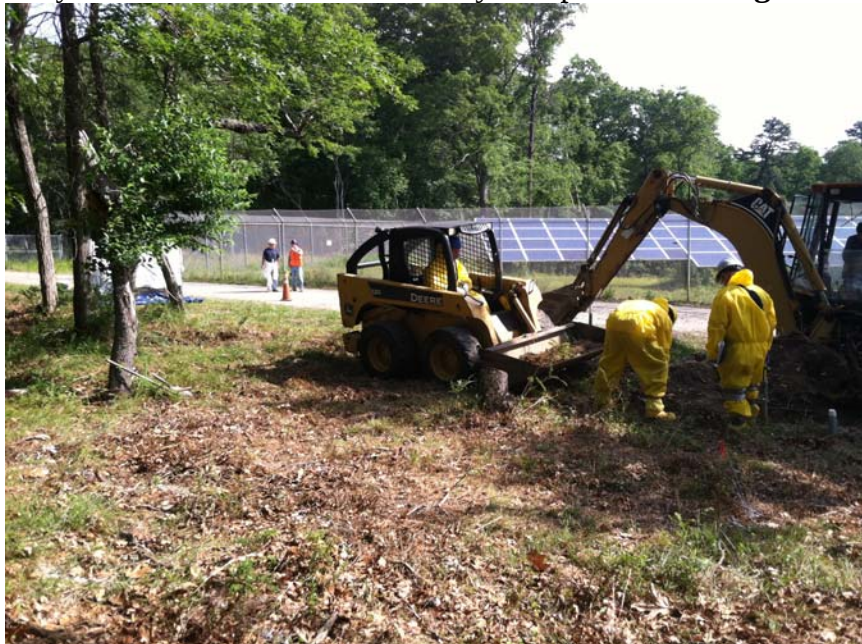
Photograph 2 – Remediation of the Phase 3 Area
