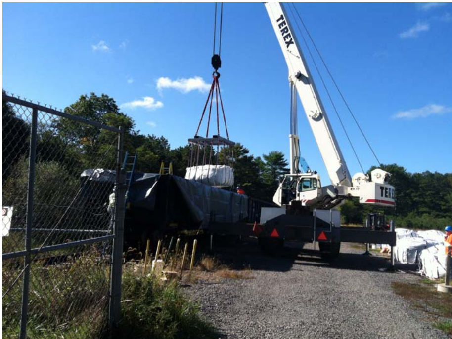
Photograph 5 – Loading Low-Sided Gondola Railcars for shipment to Energy Solutions of Utah
