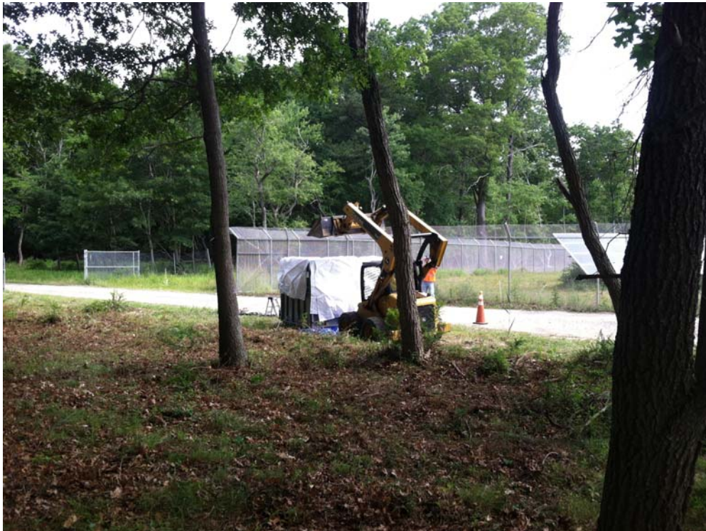
Photograph 3 – Loading Excavated Soil into a Lift Liner TM
