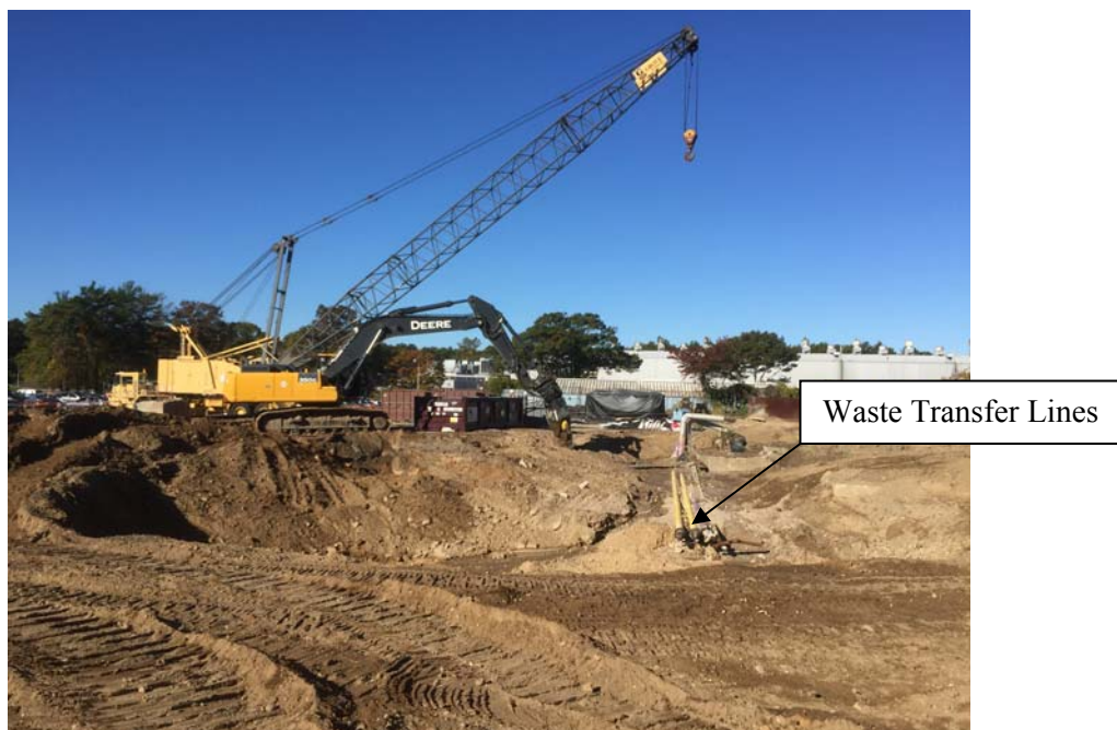
Photograph 7 – Waste Transfer Lines Removal
