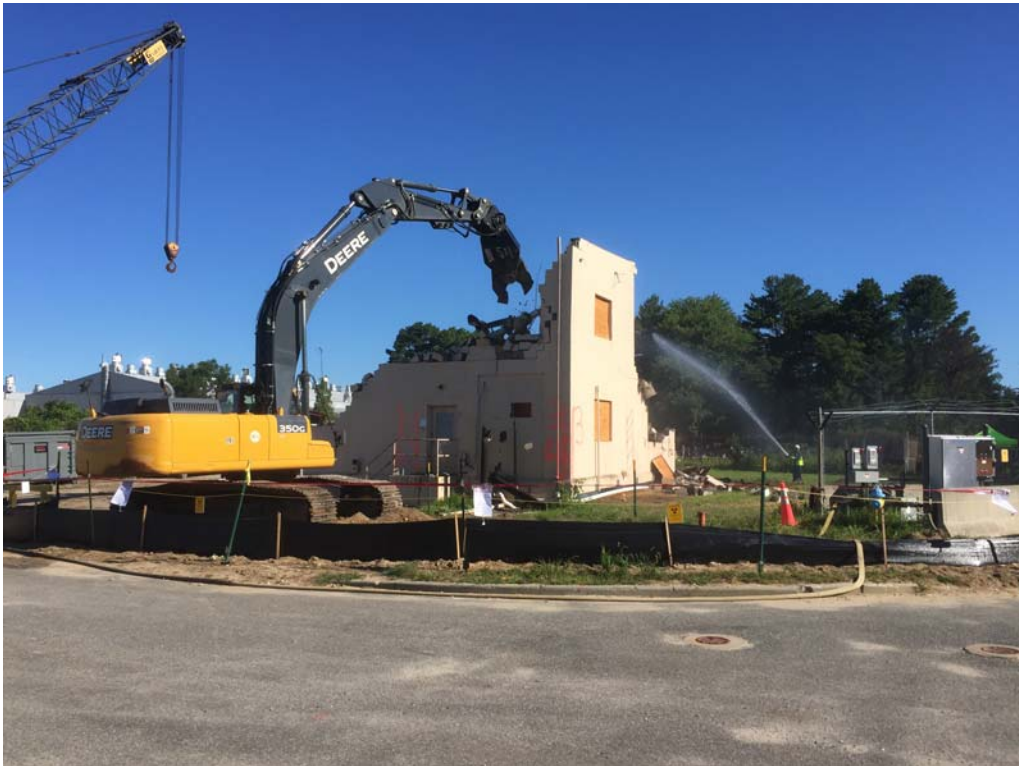
Photograph 5 – Demolition of Building 811
