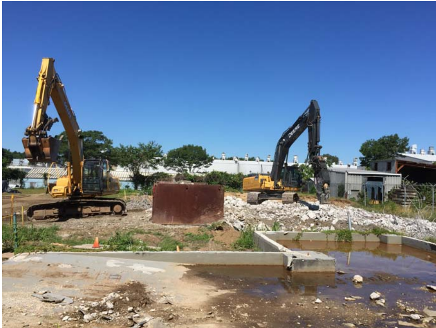
Photograph 6 – Demolition of AST Concrete Supports
