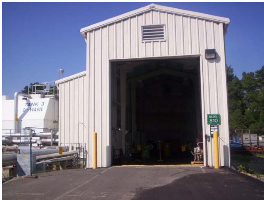
Photograph 2 – View of Building 810
