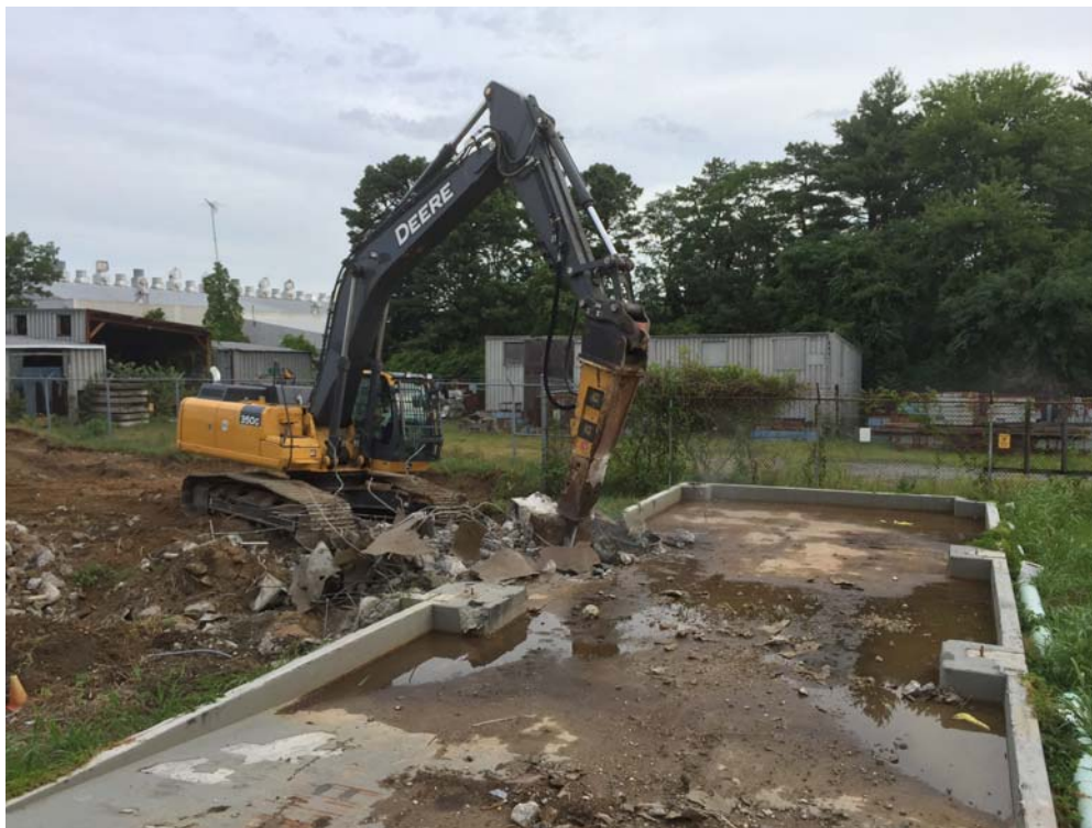
Photograph 4 – Demolition of Building 810 Foundation
