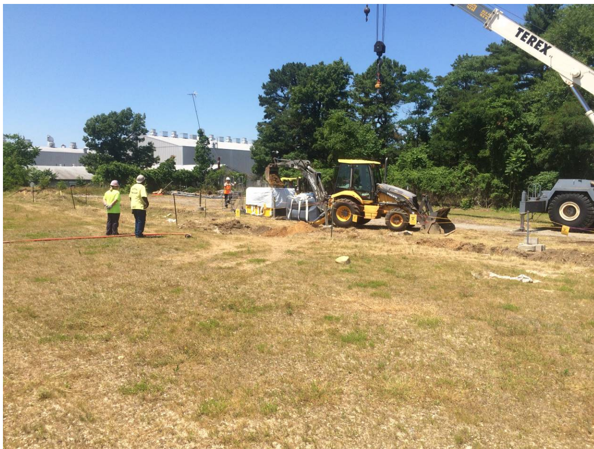
Photograph 2 – Remediation of isolated area of surface soil contamination
