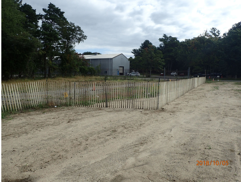
Photograph 6 – Backfilled remediated areas
