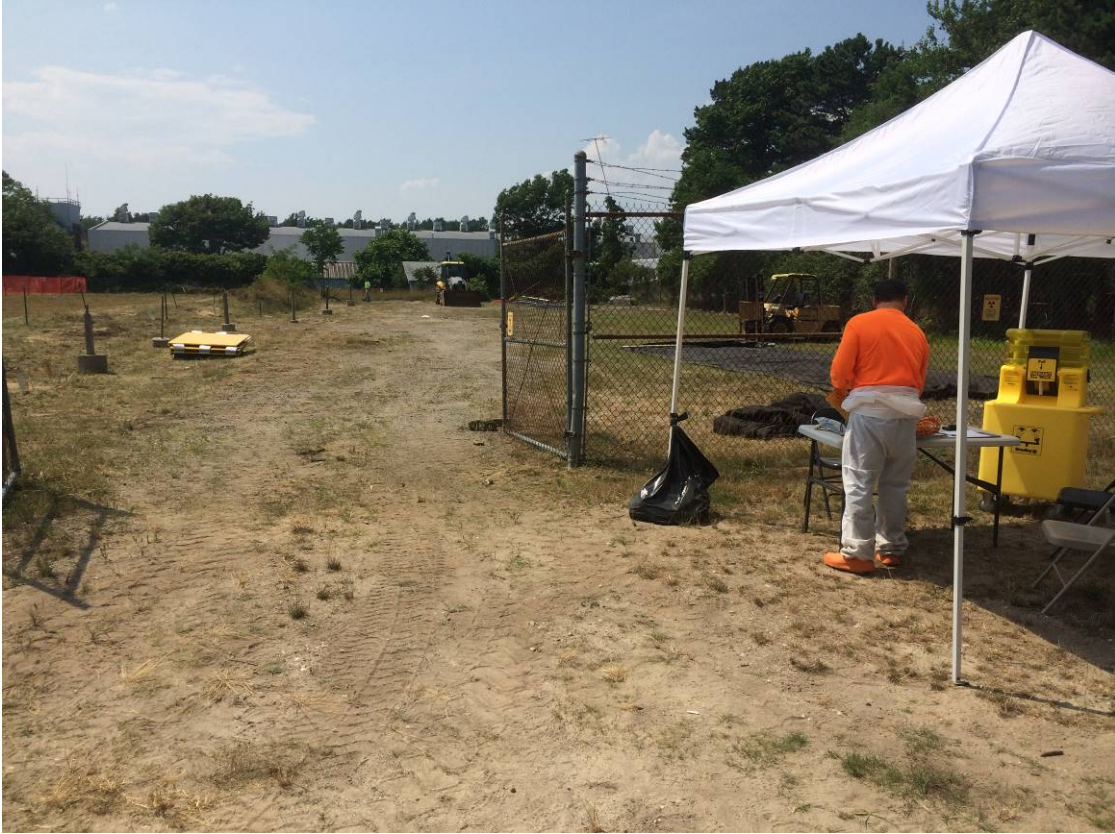
Photograph 1 – Project area, view to west
