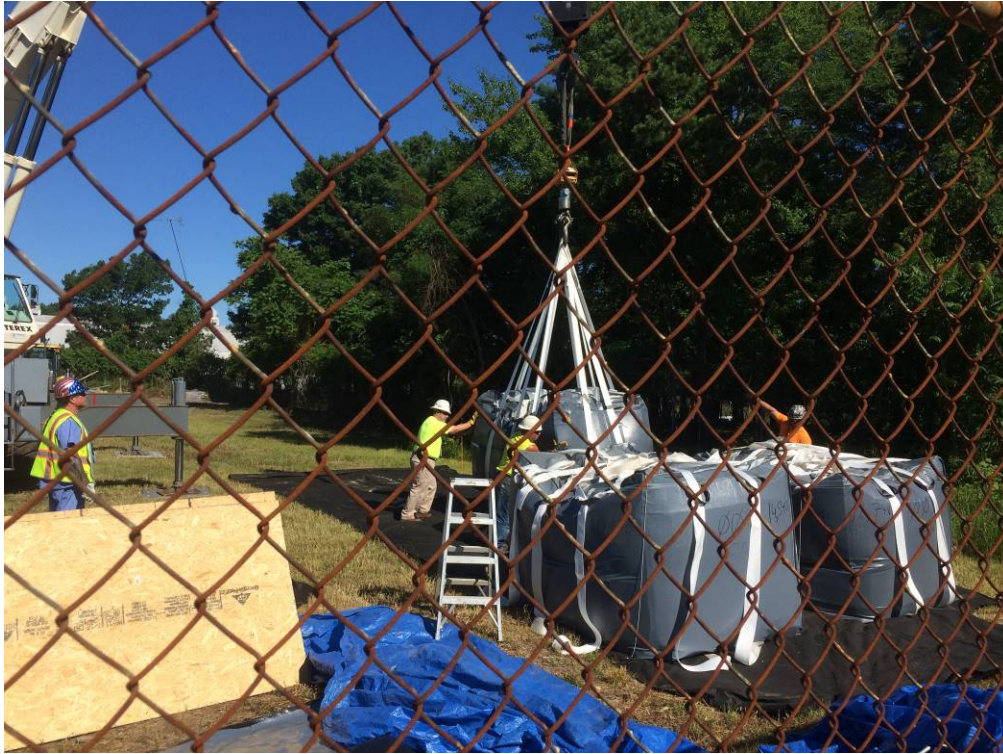
Photograph 5 – Excavated soil packaged in SPS Packaging Bags
