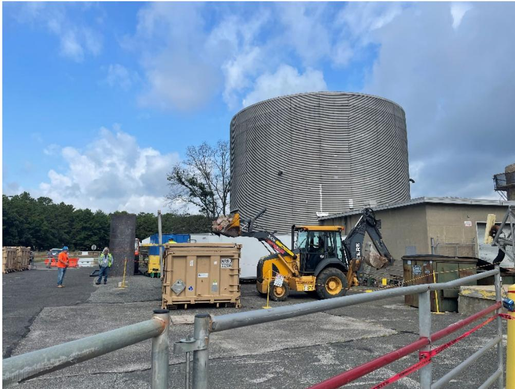
**Photograph 9 – Backhoe Loading Debris into Intermodal**
