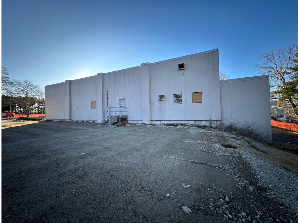
East Elevation (facing west)
