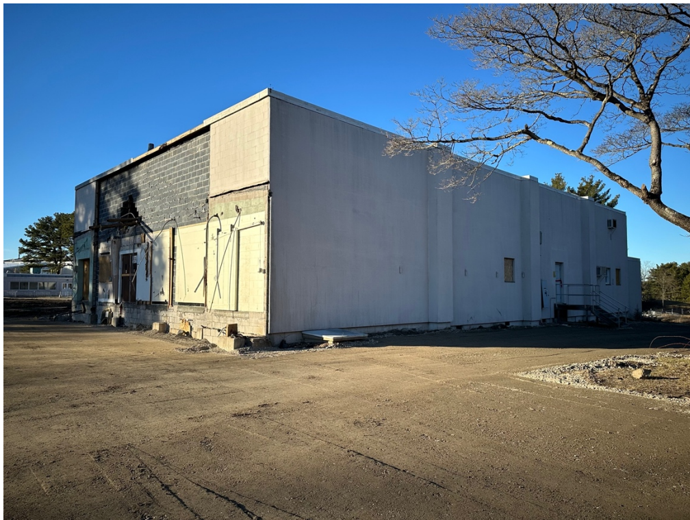
Surrounding grade has been leveled with RCA (facing northwest).
