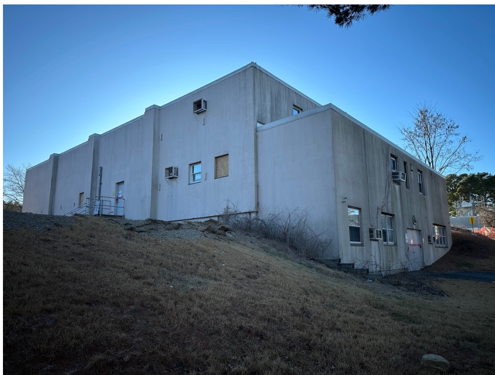
East and north side (facing southwest).
