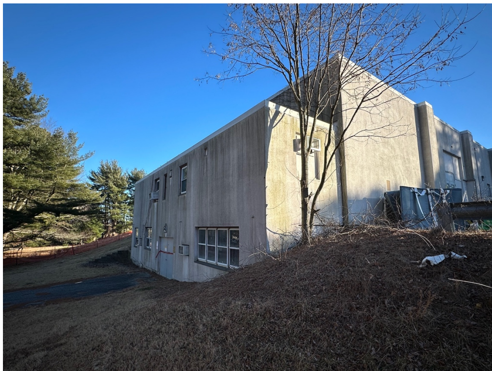
The site slopes at the rear (north) to expose the basement level (facing southeast).
