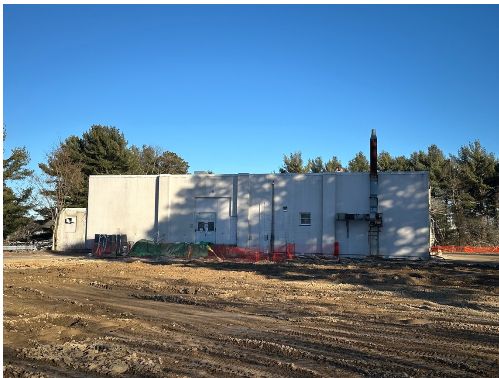
West Elevation (facing east)
