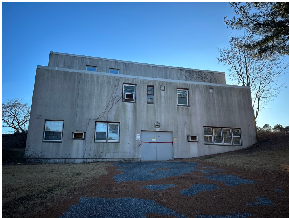
North Elevation with walk-out basement (facing south).
