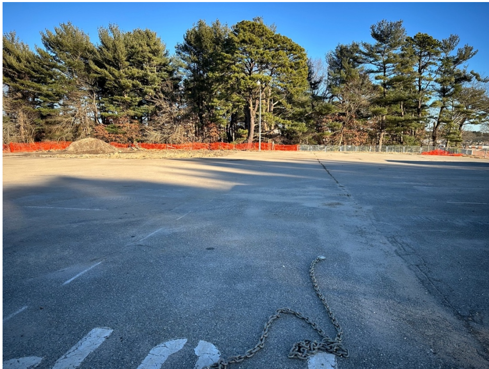
A paved staging area at the east side of the site will be outside of the regulated work area.
