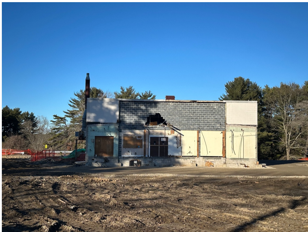
B197 High Bay Section remains. – South Elevation (facing north).
