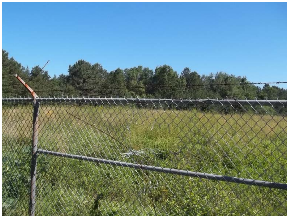
Photograph 4: Damaged fence and barbed wire at PCB capped area.
