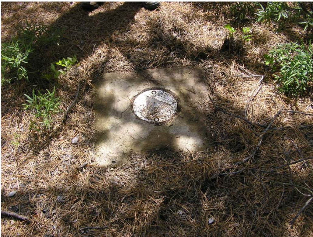
Photograph 6: Typical monitoring well prior to clearing of buffer zone.
