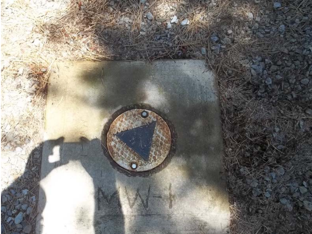
Photograph 7: Monitoring well identification in flush-mount concrete pad.
