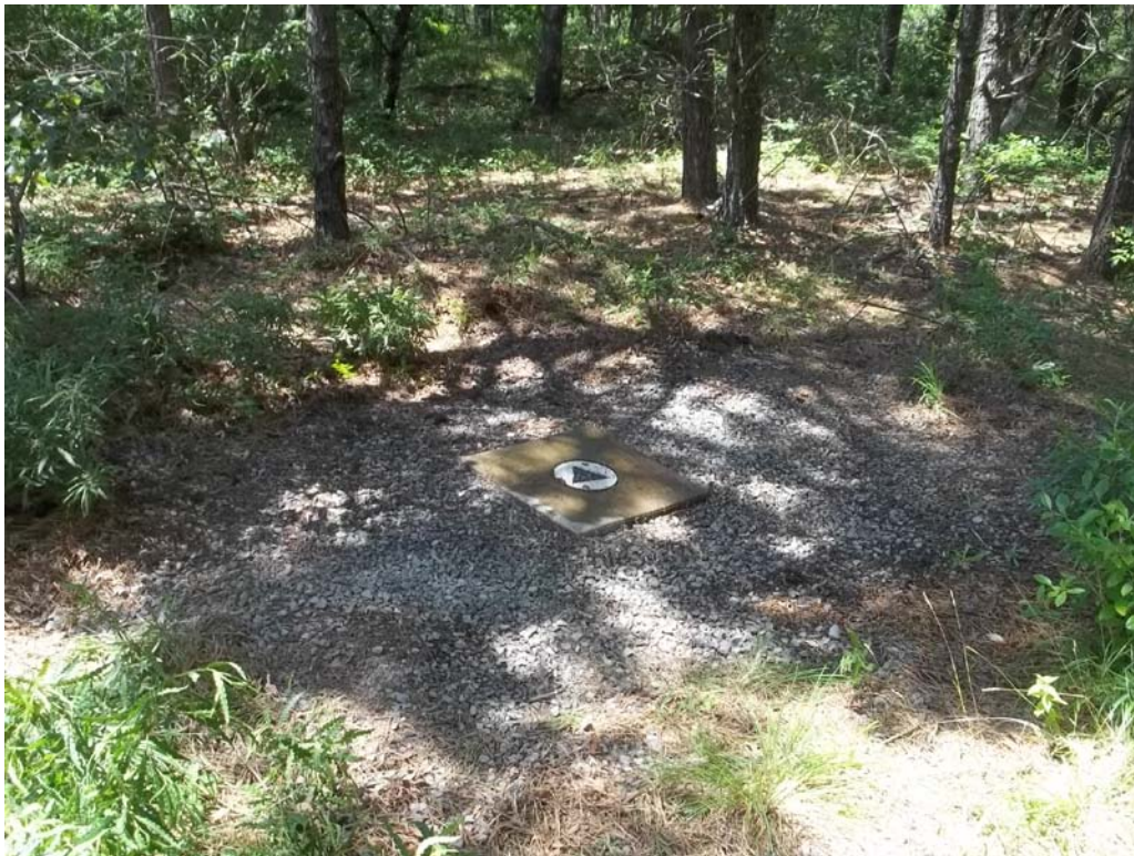
Photograph 8: Typical monitoring well following clearing of buffer zone.
