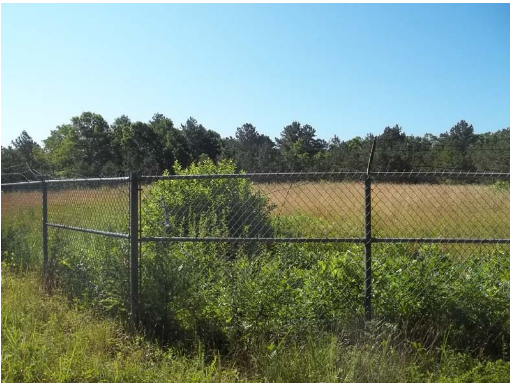
Photograph 2: Plants growing at PCB capped area and damaged barbed wire.
