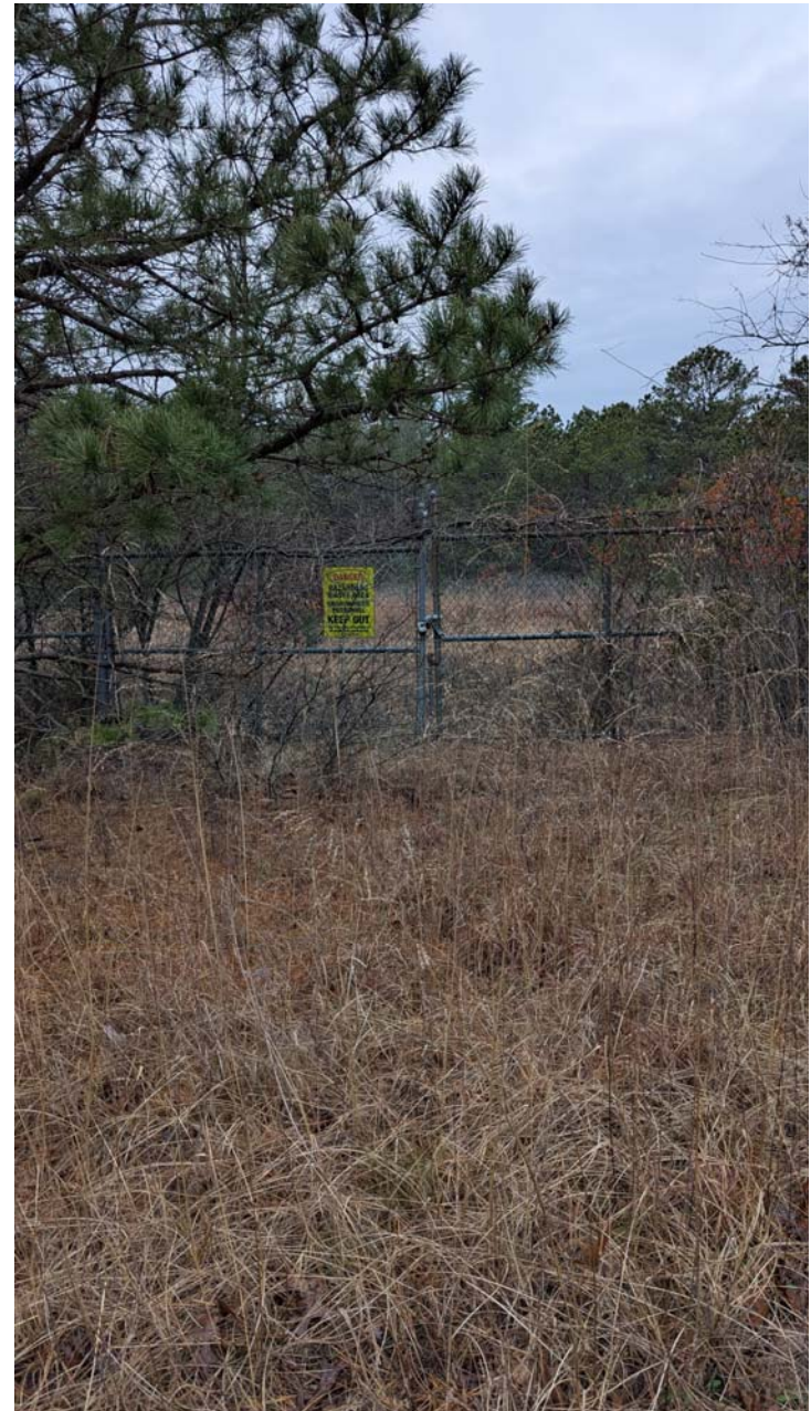
Locked fence to the Capped Area
