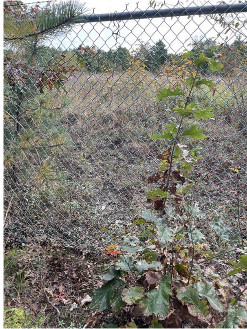
Photo 2: Repaired fencing securing Capped Area.
