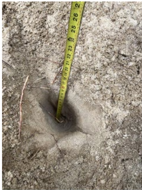
Photo 4: Manually excavated Test Pit No. 2 in Landfill Area. Sand cover verified to be at least 18 inches deep.
