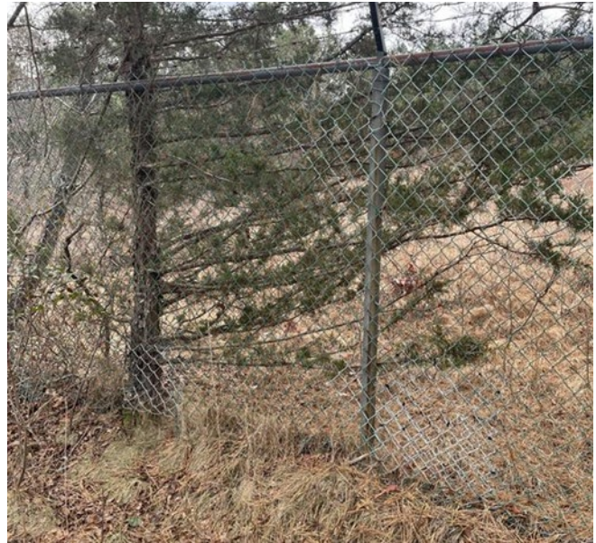
Photo 2: Repaired fencing securing Capped Area.
