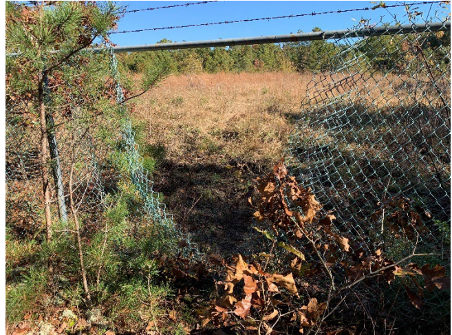
Photo 2: Hole in fencing leading to Capped Area.
