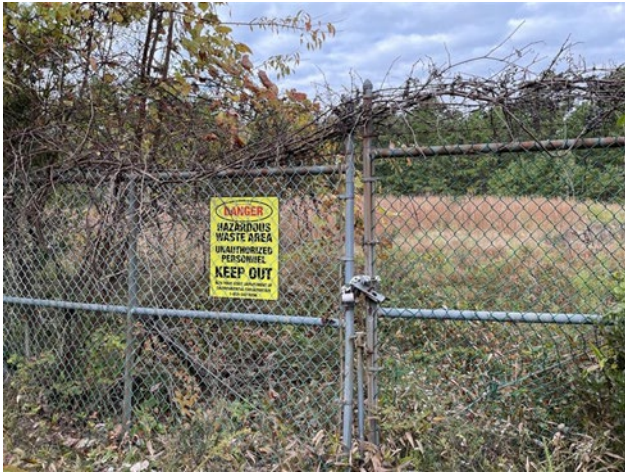
Photo 1: Access gate to the capped area is locked, however keys to locks are unavailable. "HAZARDOUS AREA" signage placed outward; no signage facing inwards.
