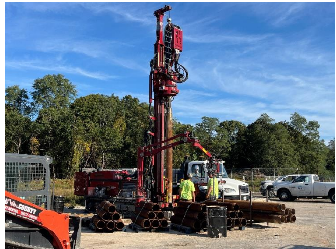
Photo 2 – Advancing 10 inch sonic casing at SB-302
