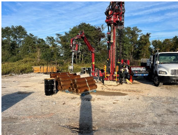
Photo 1 – 10 inch sonic casing at work area.
