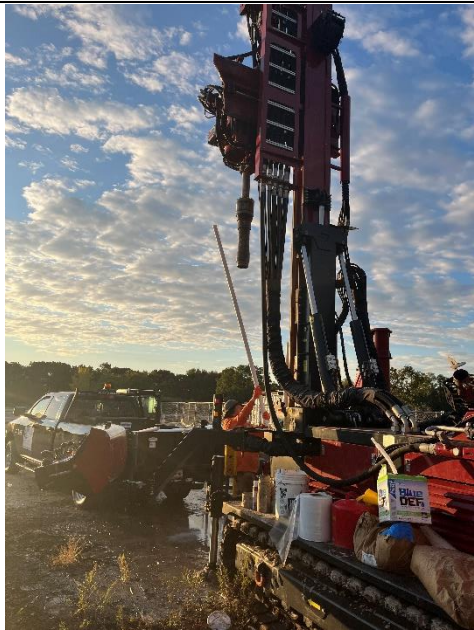
Photo 1 – PVC monitoring well installation within SB-304.
