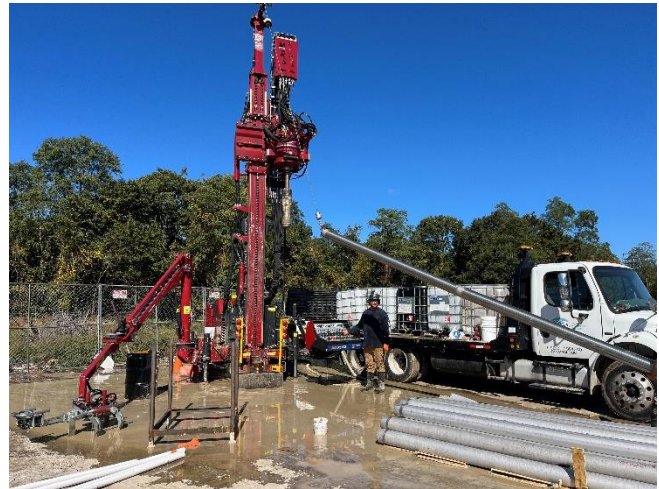
Photo 2 – Installing well HRP-IW-02 at SB-301
