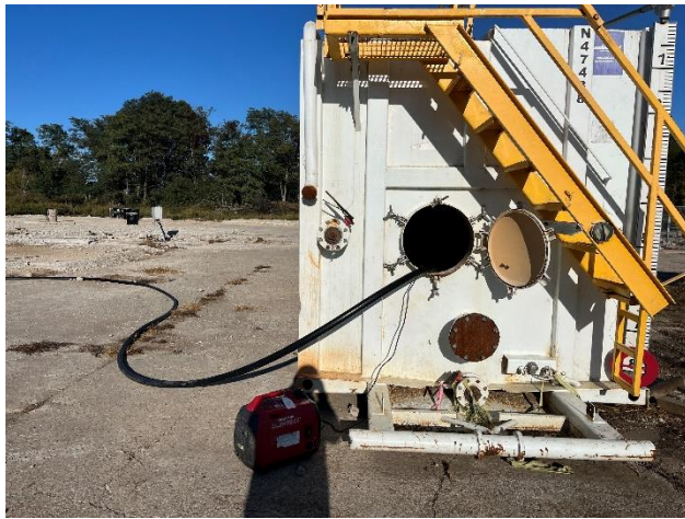
Photo 1 – Pumping from frack tank.
