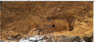
Photo 4- Single wall steel UST encountered SE of Cess-10 structure. Strong gasoline odors from inside of the tank.
