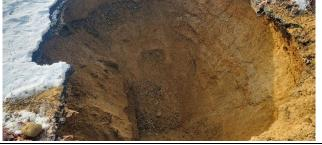
Photo 3 – Formerly backfilled cesspool structure Cess-10A was over-excavated to app. 11ft bgs and bottom was sampled.
