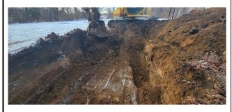
Photo 1 – Excavation of possible septic tank structure NW side of the former admin building.
