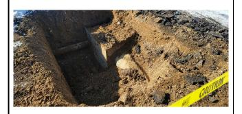
Photo 5 – Metal stormwater junction structure discovered between DW-3 and DW-4, connecting both with app. 30 inch concrete pipe.
