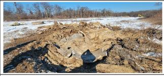
Photo 3 - Formerly backfilled septic structure Cess-2. In tact concrete cover found, structure was found to be destroyed and filled.
