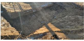
Photo 2- Top concrete cover for former septic Cess-1. No structure found, area was backfilled.
