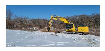
Photo 5 – Excavation and uncovering of Cess-11 septic tank at the northeast of former building "G"
