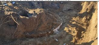
Photo 4- Uncovered septic tank Cess-12 at the north side of building "G"
