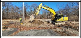
Photo 3 – Excavation of collapsed/caved in structure in front of former admin building.
