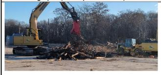
Photo 1 – Utility poles being cut into smaller sections
