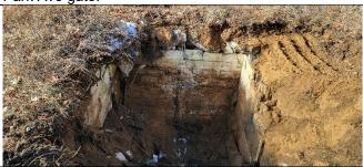
Photo 4- Uncovered cinderblock basement structure in front of admin building. Structure filled with burnt debris and concrete chunks.
