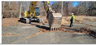
Photo 2- Excavation of an old drywell or cesspool structure in front of the admin building, close to the Park Ave gate.
