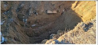
Photo 6 – Cinderblock structure with concrete roof found in front of building G. Entire structure was filled with soil.
