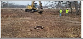
Photo 3 – Excavation and uncovering of 3 additional cesspools at the north and south of Cess-6. Pictured in the foreground is CESS-6A
