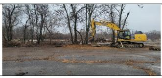
Photo 4- Excavation of tree lined area on the south side of the main parking lot where anomalies were found. No structures found.
