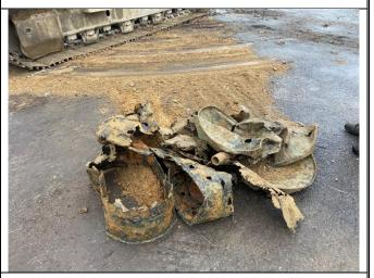
Photo 6 – Remnants of steel 55-gallon drums uncovered near CESS-11 structure.
