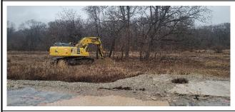
Photo 1 - Excavation of found anomaly in front of former building G.
