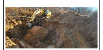
Photo 5 – Pulling of UST-3 cooling water tank. Tank shell was partially open before pull and started to peel off during removal. No staining or odors were observed in the soil beneath it.
