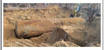
Photo 1 – Excavation of UST-2 cooling water tank at former titanium building.
