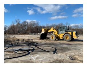
Photo 6 – RCA capping of former Cess-3 and Cess-3A locations.
